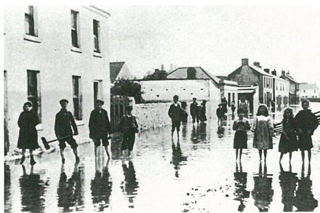
A street in Little Bray, Co. Wicklow after the flood of 25th August 1905. (Note the 'tidemark' on the wall of the houses). Similar severe flooding occurred on the same day of August 1986. (Photo: R.M. Barrington, from British Rainfall, 1905)
