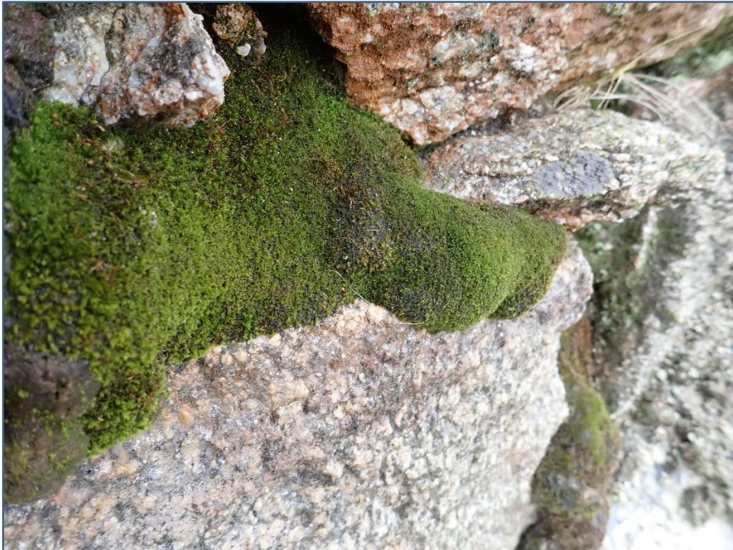
Figure 22 Cushion of Cephaloziella cf. nicholsonii on retaining wall.
