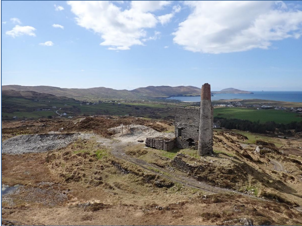
Figure 131 Overview of mine north-east of Caminches, with a small area of spoil adjacent to a well-preserved engine house.
