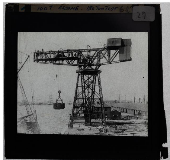
Sample from the collection showing a 100-ton crane undergoing a test – please watch the website for the appearance of captions (LS_029)
