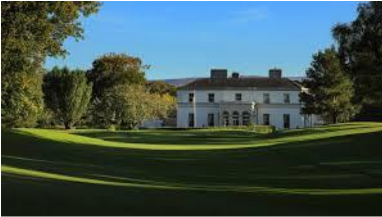
Figure 9. Tulfarris House, Co Wicklow.
