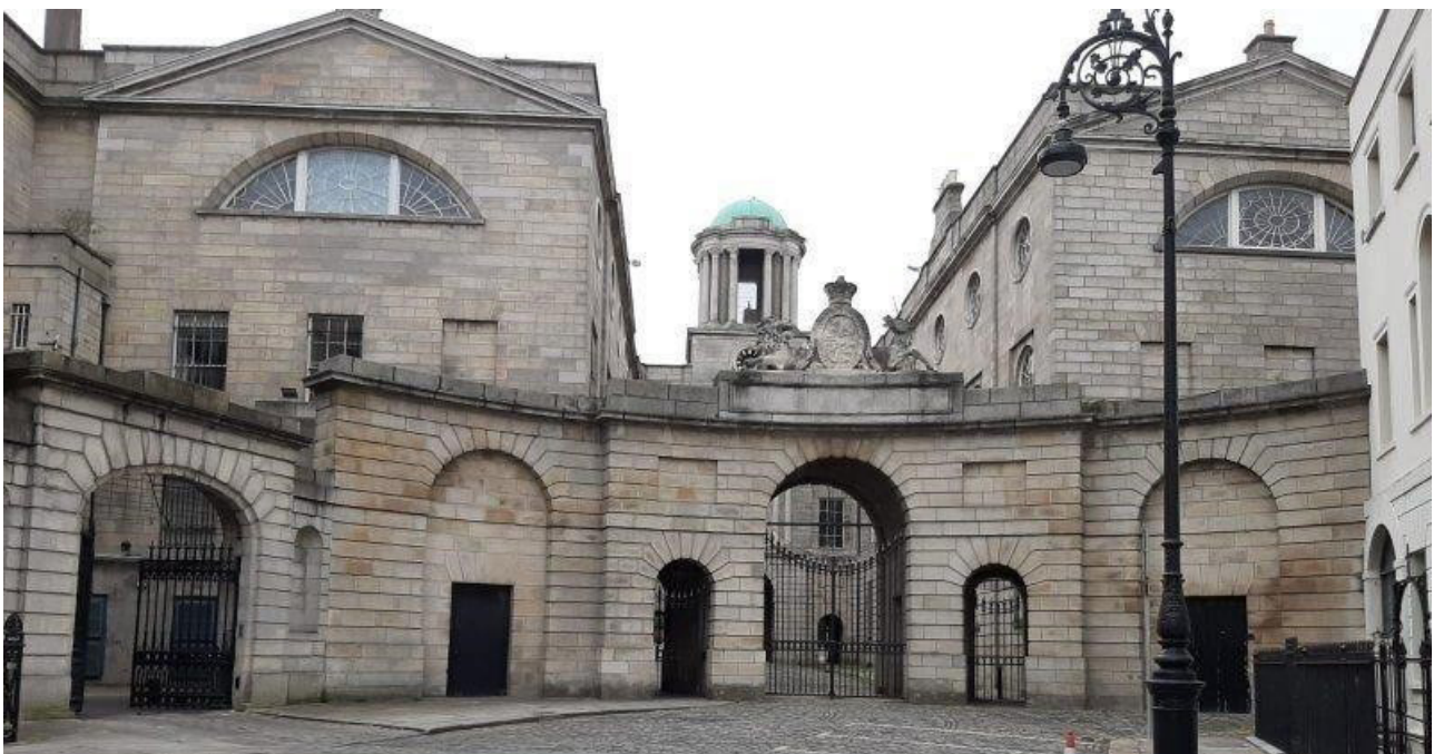
Henrietta Street entrance to Registry of Deeds and King's Inn, showing triumphal arch designed by Francis Johnston, c.1817
