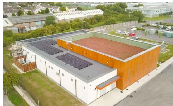
Aerial view of building with green roof on repository and solar panels on office accommodation
