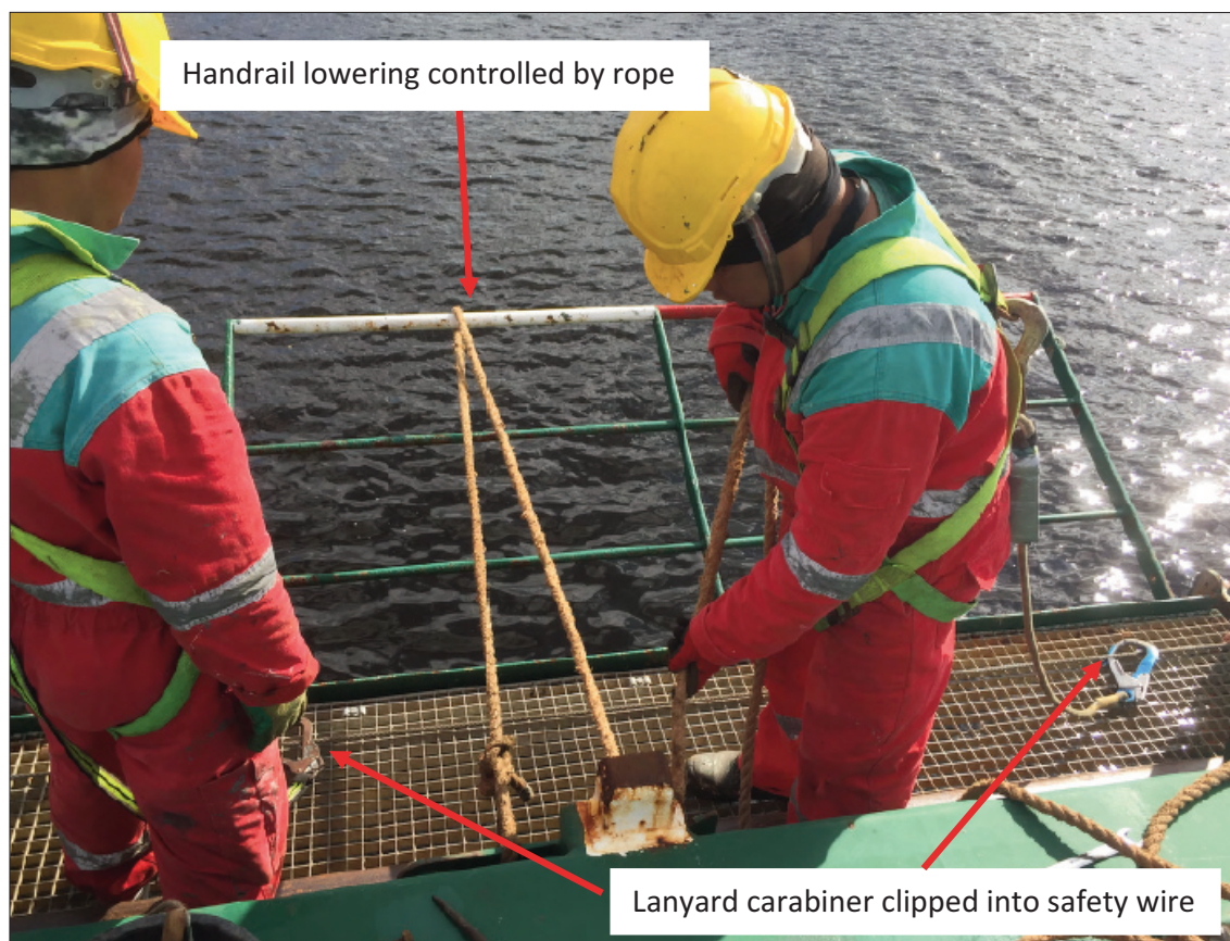
Photograph No. 2 - The Correct Method for Lowering Handrails
