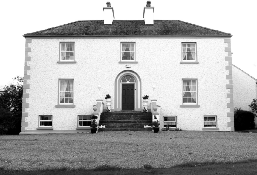
1.3 A typical glebe house near Terryglass, Co. Tipperary (image reproduced courtesy of the NIAH).
