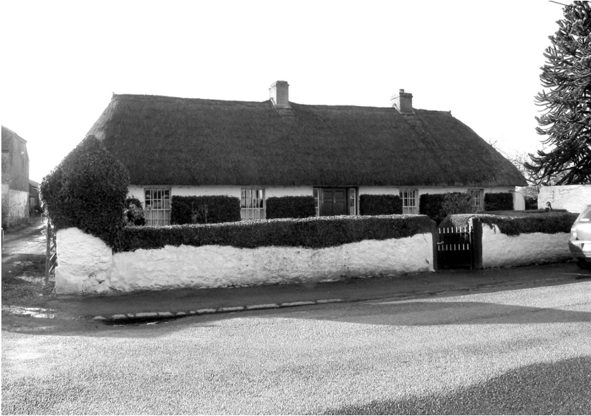
1.1 Abbeyview Cottage, Co. Laois (photograph by the author, with thanks to Michael Dempsey).
