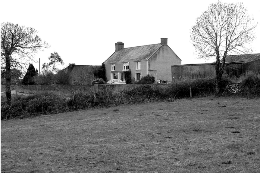
1.5 Shannon Hall, Co. Tipperary, with remodelled windows (image reproduced courtesy of Peter Clarke).
