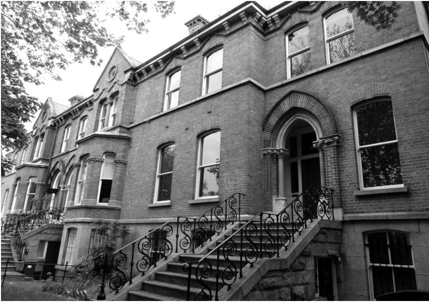
2.6 Nos 46–52 Northumberland Road, Dublin (photograph by the author).
