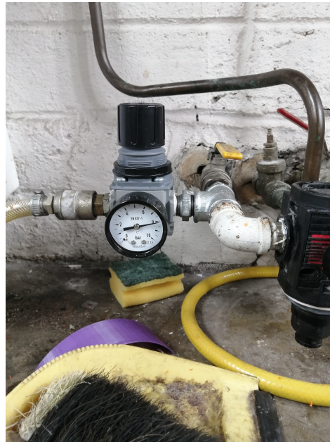
Figure A.1: Valve under the sink (open), allowing the compressed air tank to fill up
