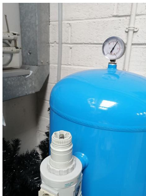
Figure A.2: Tank valve (open), allowing the compressed air to flow in the system
