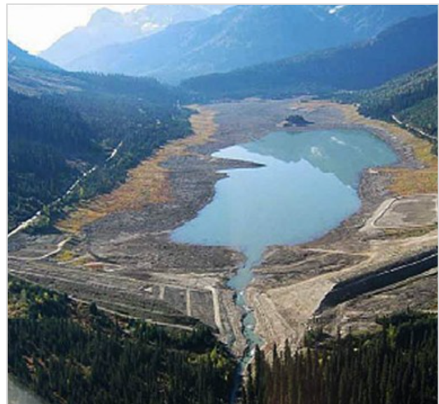
Figure 4. Coursier Lake Dam and reservoir after decommissioning (courtesy BC Hydro).
