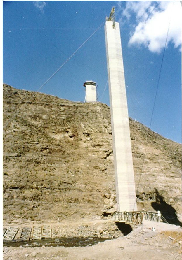
Figure 3. Pier K Foundation, Malibamatso River Bridge, Lesotho. (Hartford, 1994).
