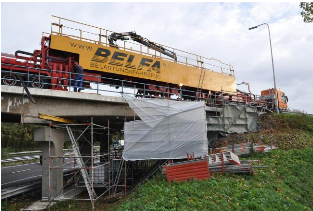
Figure 1: The German BELFA load testing vehicle on viaduct Vlijmen-Oost in The Netherlands. Reprinted with permission from (Lantsoght et al. 2017).
