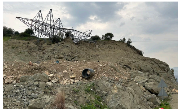
Figure 1. Earthquake-induced landslide causing differential displacement of the legs of an electric transmission tower and collapse, from the 2023 M7.8 Kahramanmaraş Earthquake.
