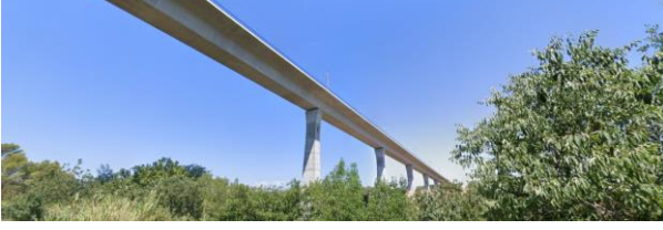
Figure 2: Multi-span railway bridge in Spain.
