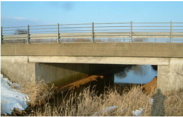
Figure 3: Bridge passing Heager Å. Photo taken from (Generaleftersynsrapport, (2006)).
