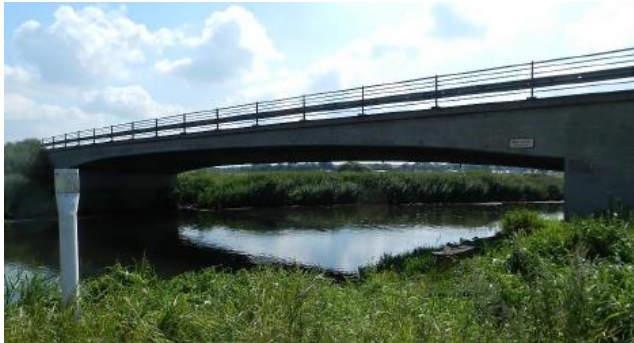
Figure 5: Bridge passing Ribe Vester Å Photo taken from (Generaleftersynsrapport, (2014)).
