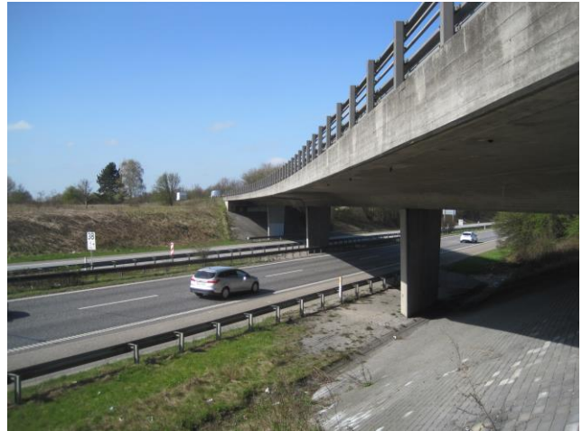
Figure 9: Bridge passing Vestmotorvejen.
