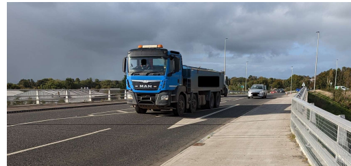
Figure 6: An HGV lorry that caused acceleration response of the bridge deck similar to the response seen in Figure 5.
