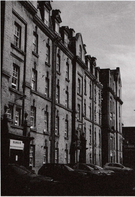
5 Kevin Street flats, Dublin, 1894–1901, R.J. Stirling for the Guinness Trust. Photo: L. King (2012).
