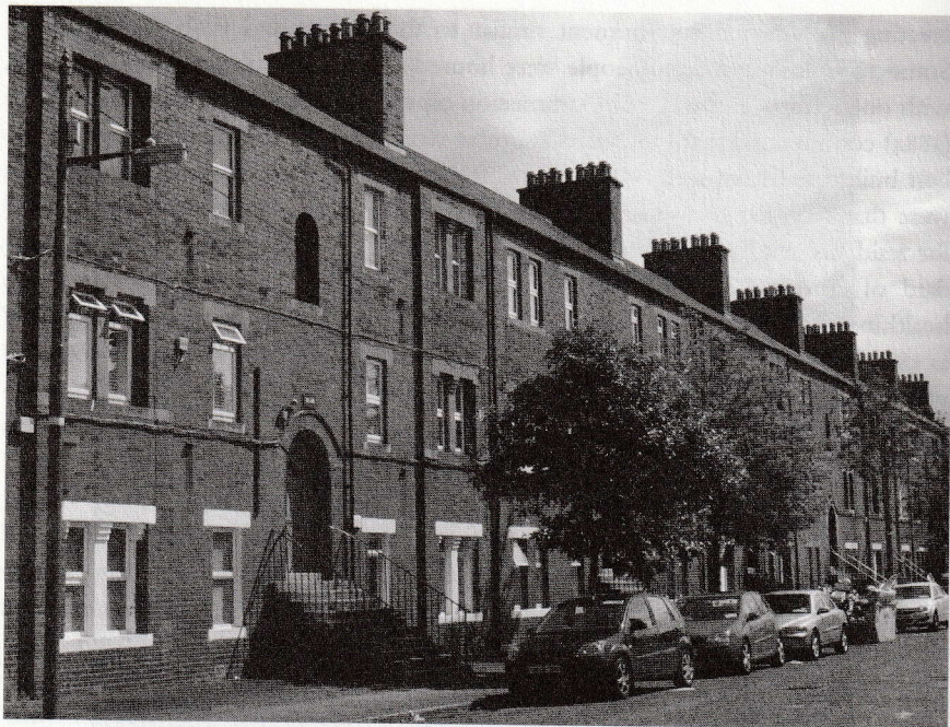
3 Rialto Buildings, Dublin, 1883, C.H. Ashworth for Guinness Brewery. Photo: L. King (2012).
