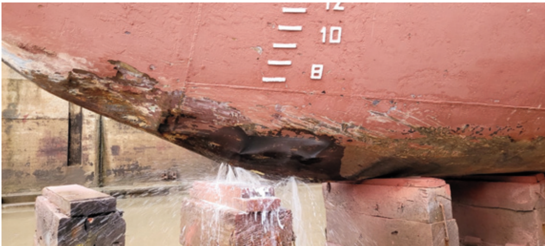
Forepeak bottom damage to Arklow Raider
