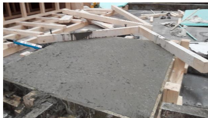
Figure 4-13 Completed trial slab
