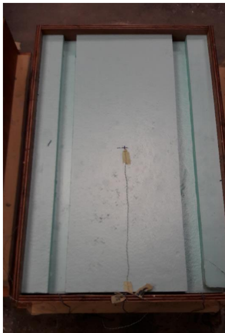
Figure 5-4 Control panel prior to HPFRC layer being poured with thermocouple in place
