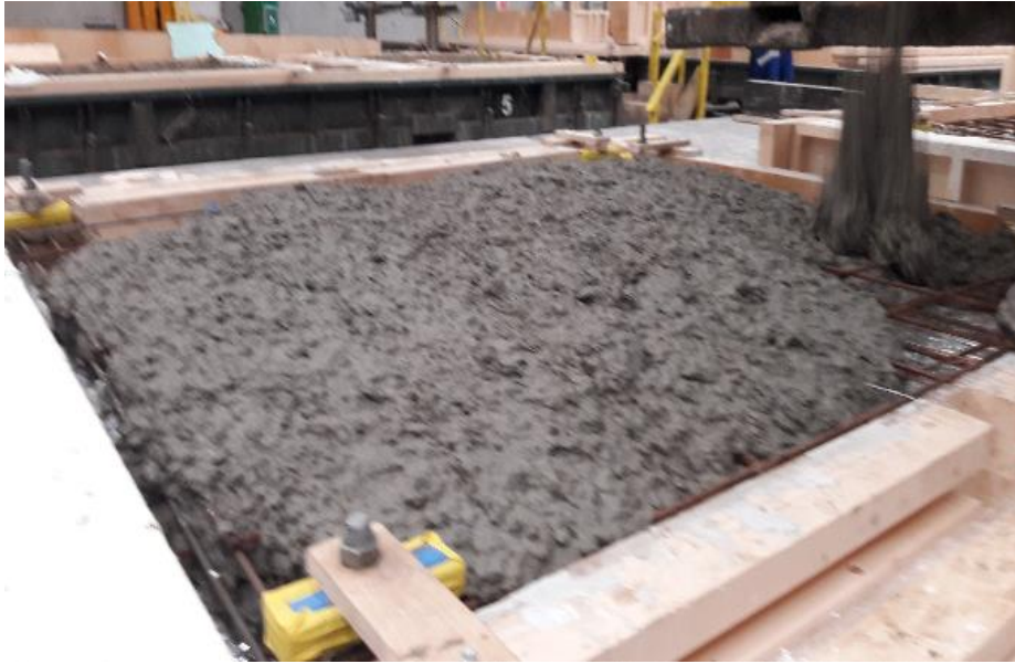
Figure 7-11 Placement of fresh PCM-concrete composite into the panel
