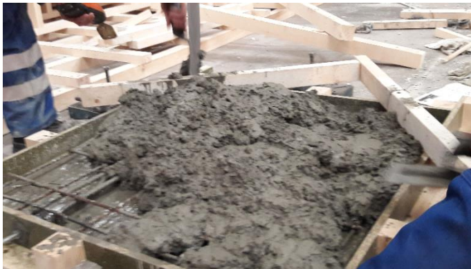
Figure 4-12 PCM-concrete being poured
