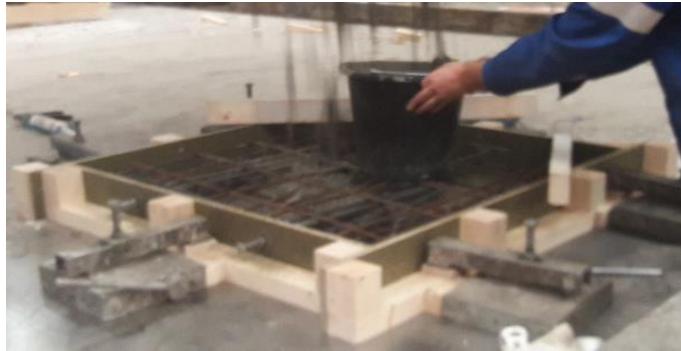
Figure 4-11 60 mm layer of control mix being poured
