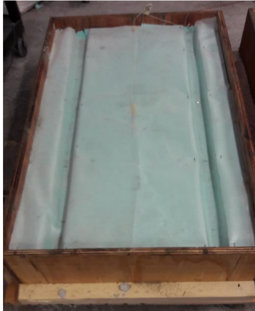
Figure 6-1 Control debonded panel with debonding sheet prior to pouring the outer HPFRC wythe
