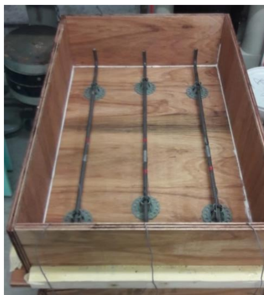
Figure 5-2 Formwork and reinforcement for panels
