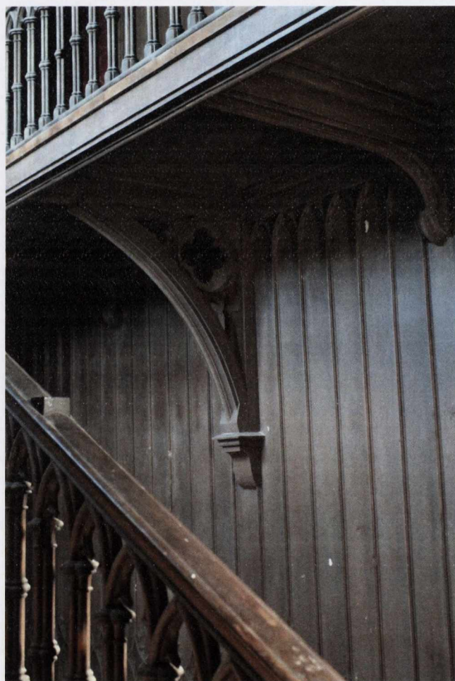
Fig. 3.92 Charleville Castle, detail of walls to main staircase and supports for balcony, Francis Johnston, built 1804–1805, photograph Judith Hill, 2016.
