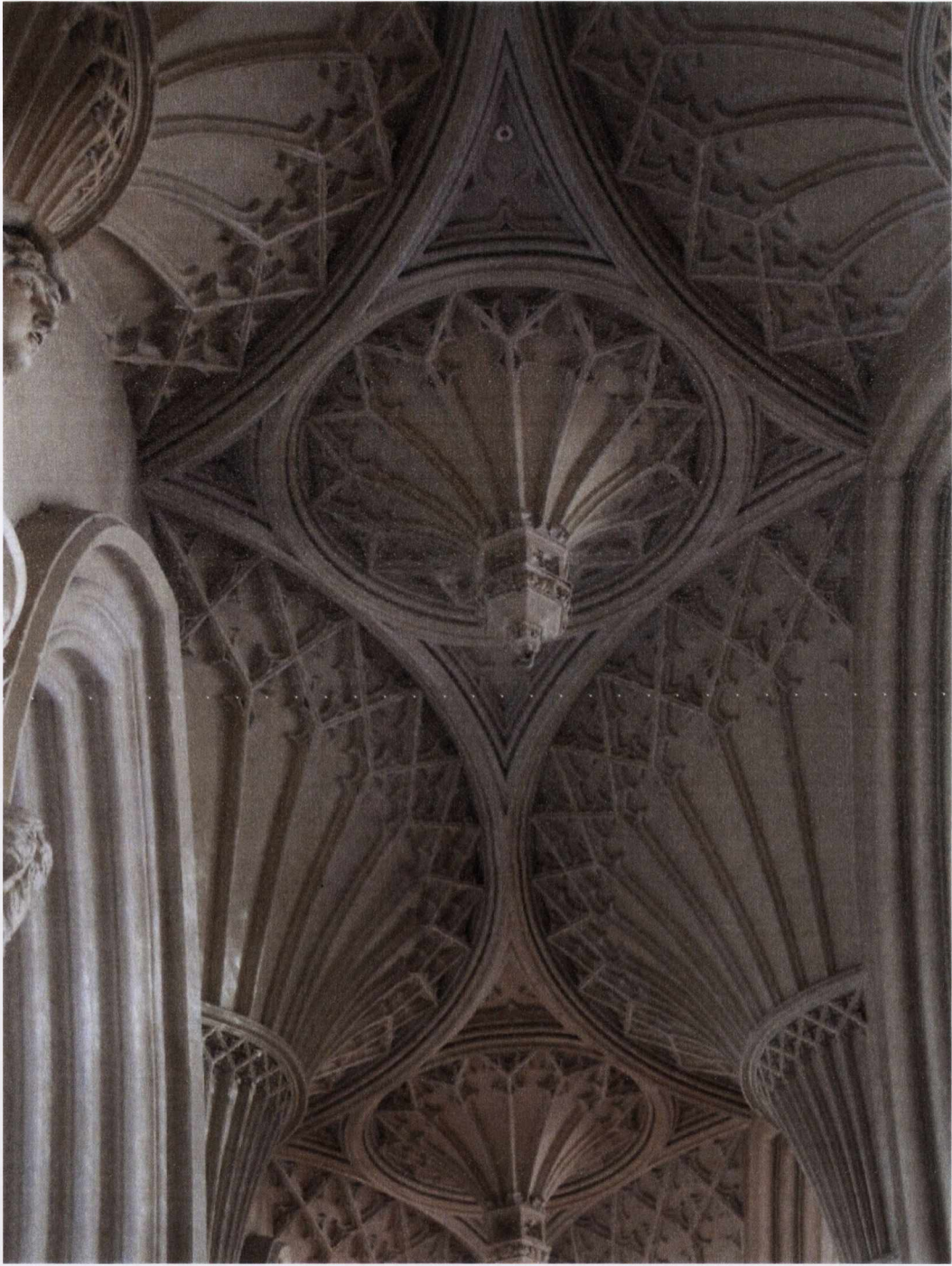
Fig. 5.23 Castle Chapel, Dublin Castle, Gallery fan vaulting, George Stapleton, modelled 1811–1812, photograph Judith Hill. 2014.
