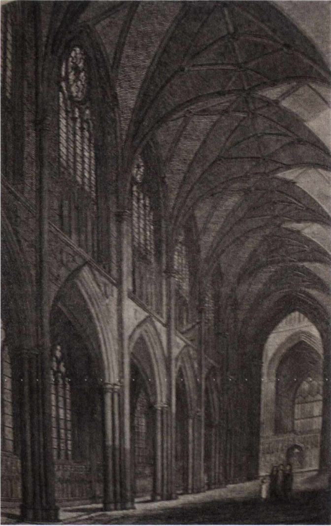
Fig. 2.30 'Interior view of the nave of York Minster', from Milner, A treatise on the ecclesiastical architecture of England (1806–11), pl. 9, RIBA Collections.
