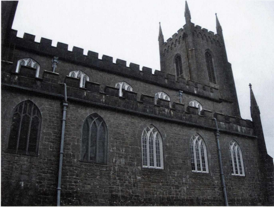
Fig. 3.104 Church, Tullamore, Francis Johnston, constructed 1808–1815, photograph Judith Hill, 2013.
