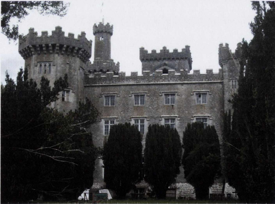
Fig. 3.79 Charleville Castle, view of west elevation, constructed 1801–1804, photograph Judith Hill, 2012.
