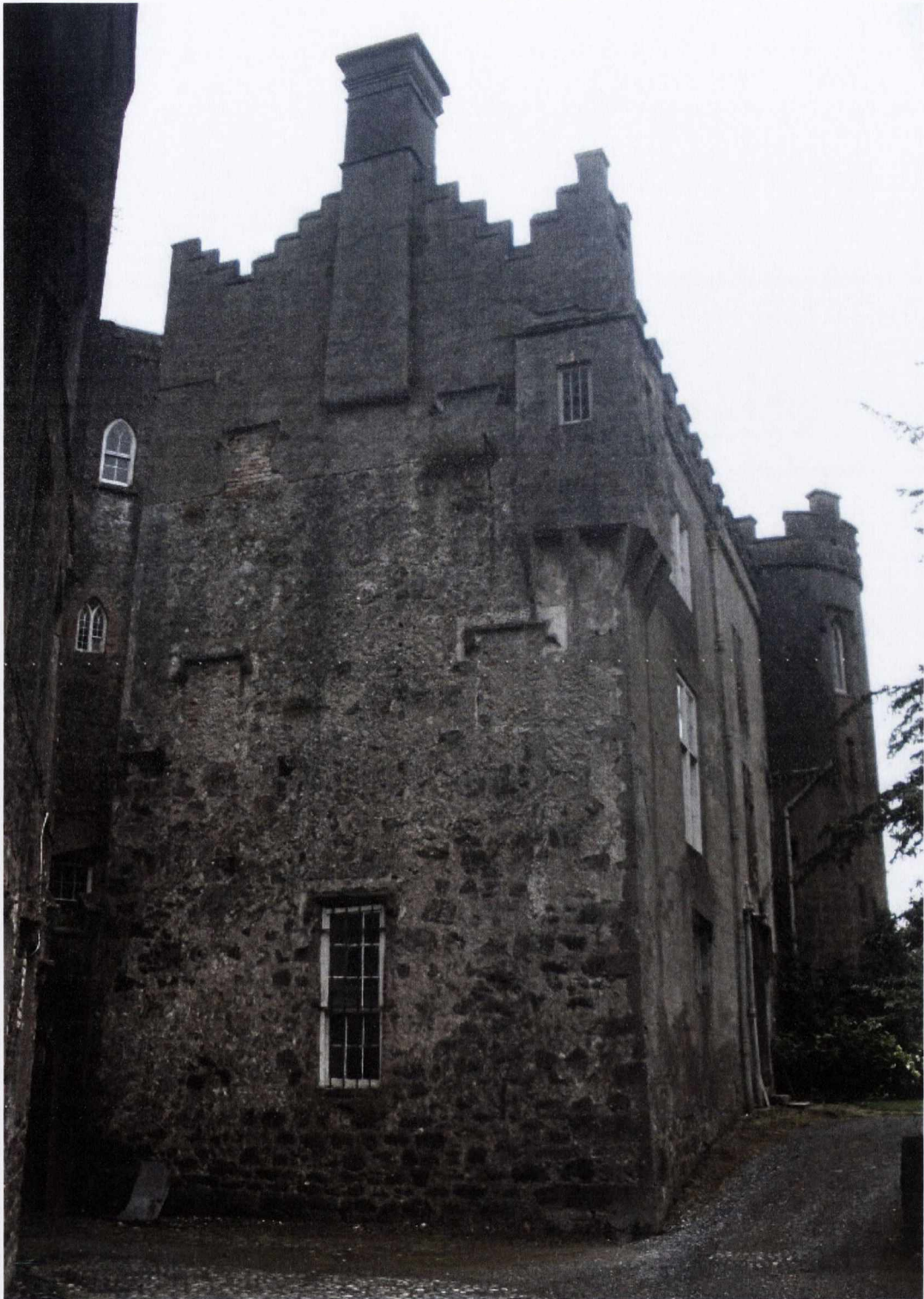
Fig. 4.15 Birr Castle, south-east elevation of the east flanker showing seventeenth-century bartizan, photograph Judith Hill, 2013.
