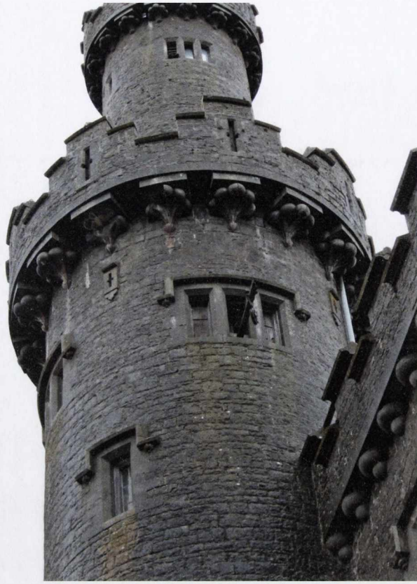
Fig. 3.74 Charleville Castle, north elevation, detail of corbelling on round tower and under battlements, Francis Johnston, constructed 1801–1804, photograph Judith Hill, 2016.
