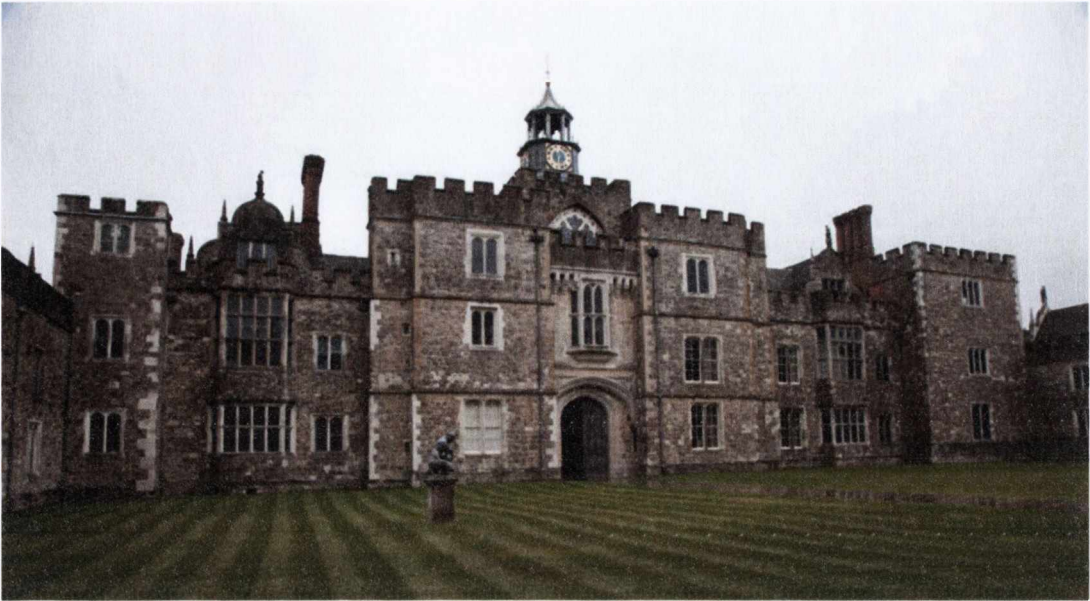
Fig. 4.32 Knole, Sevenoaks, Kent, elevation of east range, photograph www.taylorjyoungphotography.com
