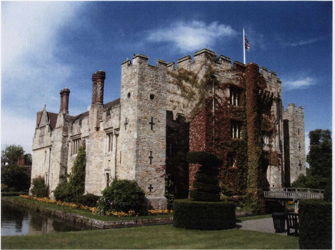
Fig. 4.30 Hever Castle, Sevenoaks, Kent, south elevation of, photograph from Wikipedia, en.wikipedia.org .
