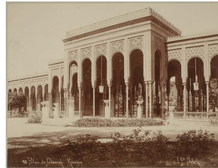
Fig. 5 J. Pascal Sébah (1823–86), Historic View of the Gezira Palace Kiosk Facade , Cairo (now destroyed), 1870s. Albumen print. Courtesy of Special Collections, Fine Arts Library, Harvard University.
