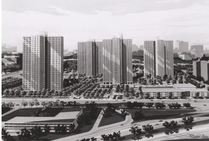
(a) Polo Ground Towers
