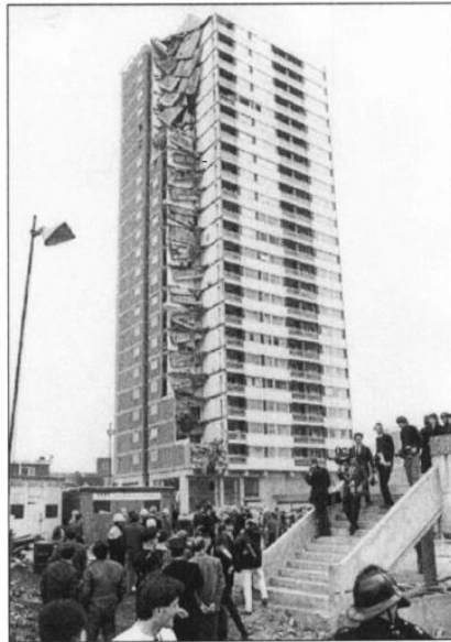
Figure 1: Ronan Point apartment tower after collapse.
