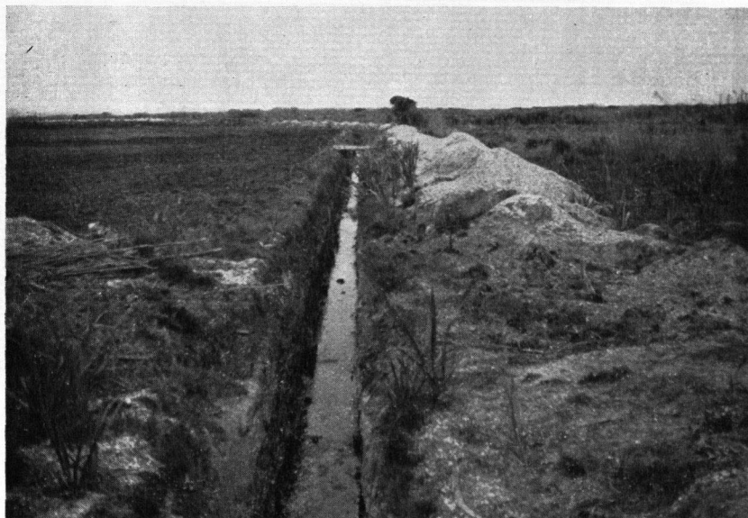
PLATE 3.—Land development, Seaward Moss, at the extreme south of the South Island. Here, with peaty soils, difficult to drain, and a cool, damp climate, conditions are not dissimilar to those found widely in Ireland. On the left, cultivated land drained by the 6-foot deep channel; on the right, the original marsh and scrub vegetation.
