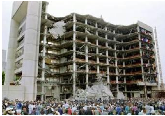
Figure 6.4 Murrah Building after the bombing
