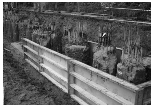
(b) Placement of formwork for capping beam.
