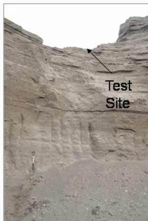
Figure 2. Excavations at Blessington test site (after [4]).
