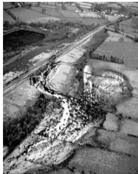
Figure 2 - Canal embankment failure at Edenderry (Pigott et al. 1992).
