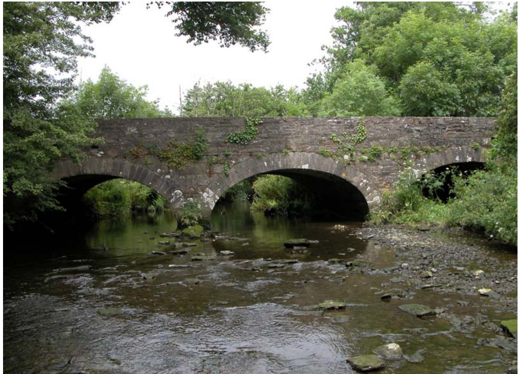
Belgooly Bridge on the Stick River (W663537) – 07 July 2005 – M.Bailey
