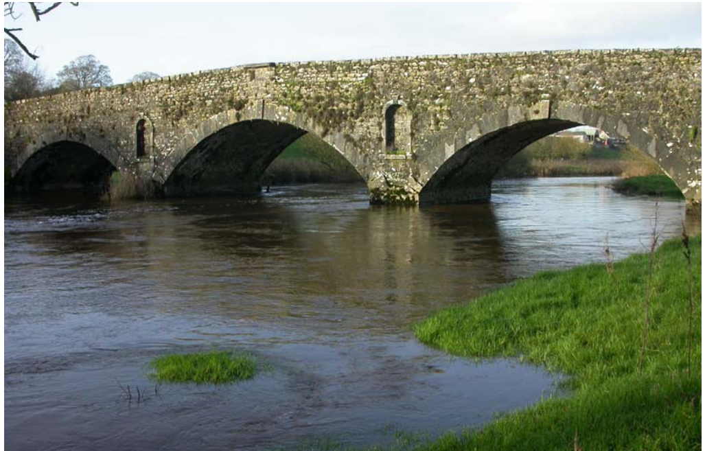
Threecastles Bridge on the River Nore (S458627) – 11 Jan 2005 – M.Bailey
