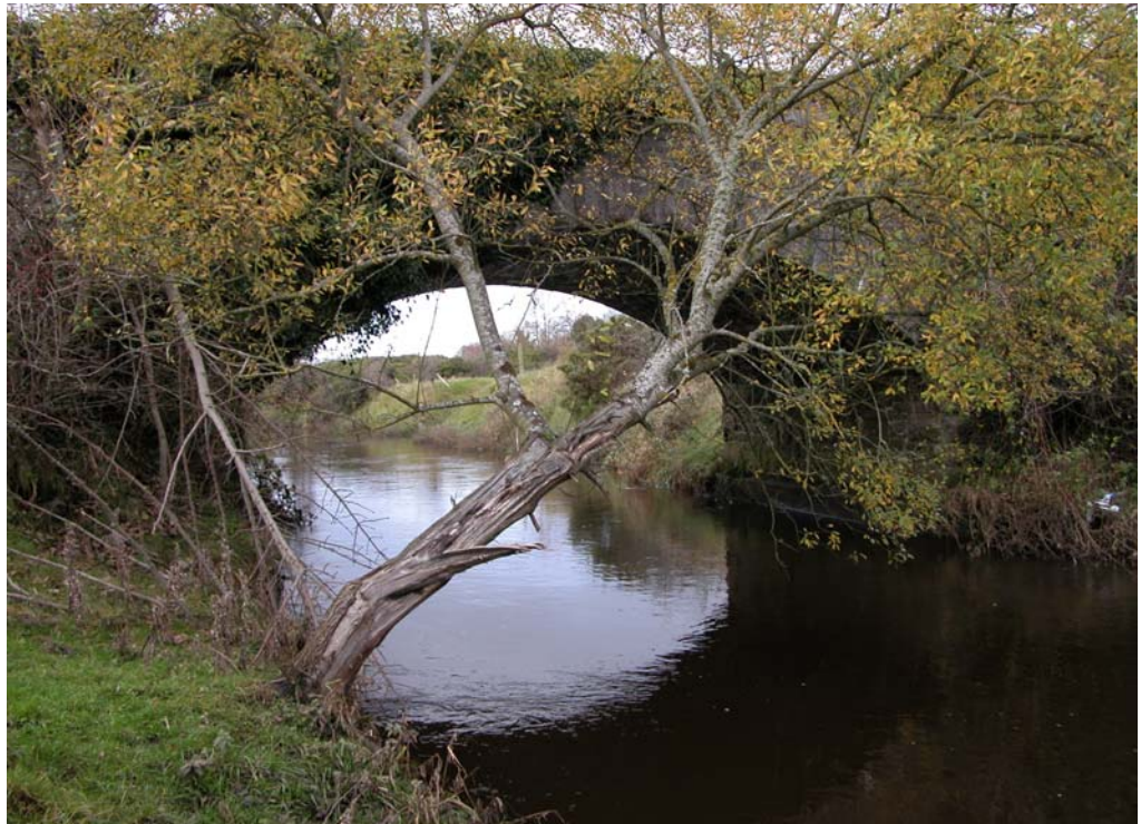
Scarriff Bridge on the Stonyford River (N732533) – 22 Nov 2004 – M.Bailey
