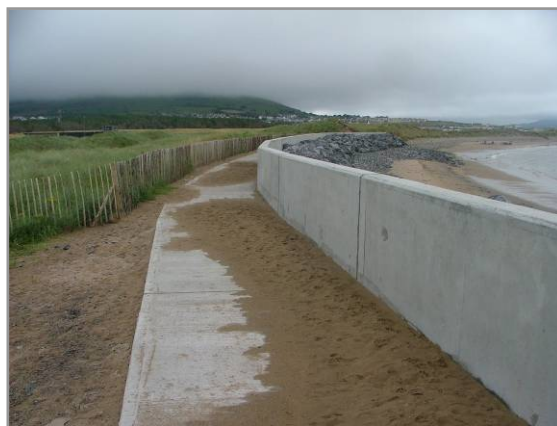
Figure 4.1: Sea wall and rock armour at site 133 Strandhill, Co. Sligo.
