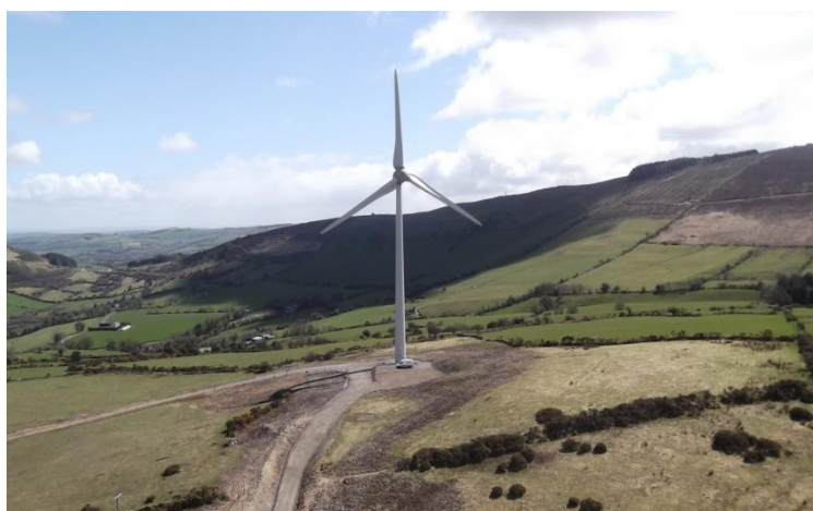
Figure 4.4 ENERCON E-70 at Templederry Wind Farm
