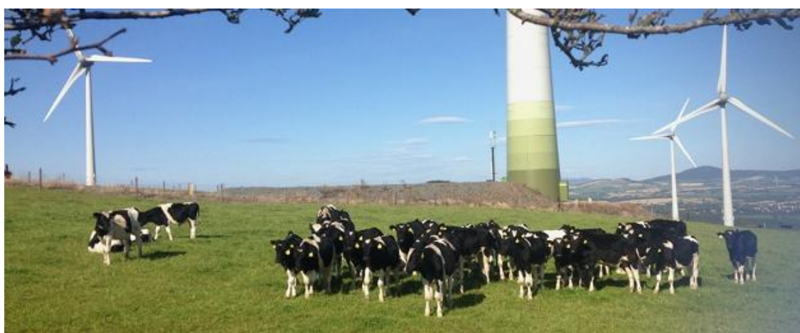
Figure 4.11 Castledockerell Wind Farm, Bunclody
