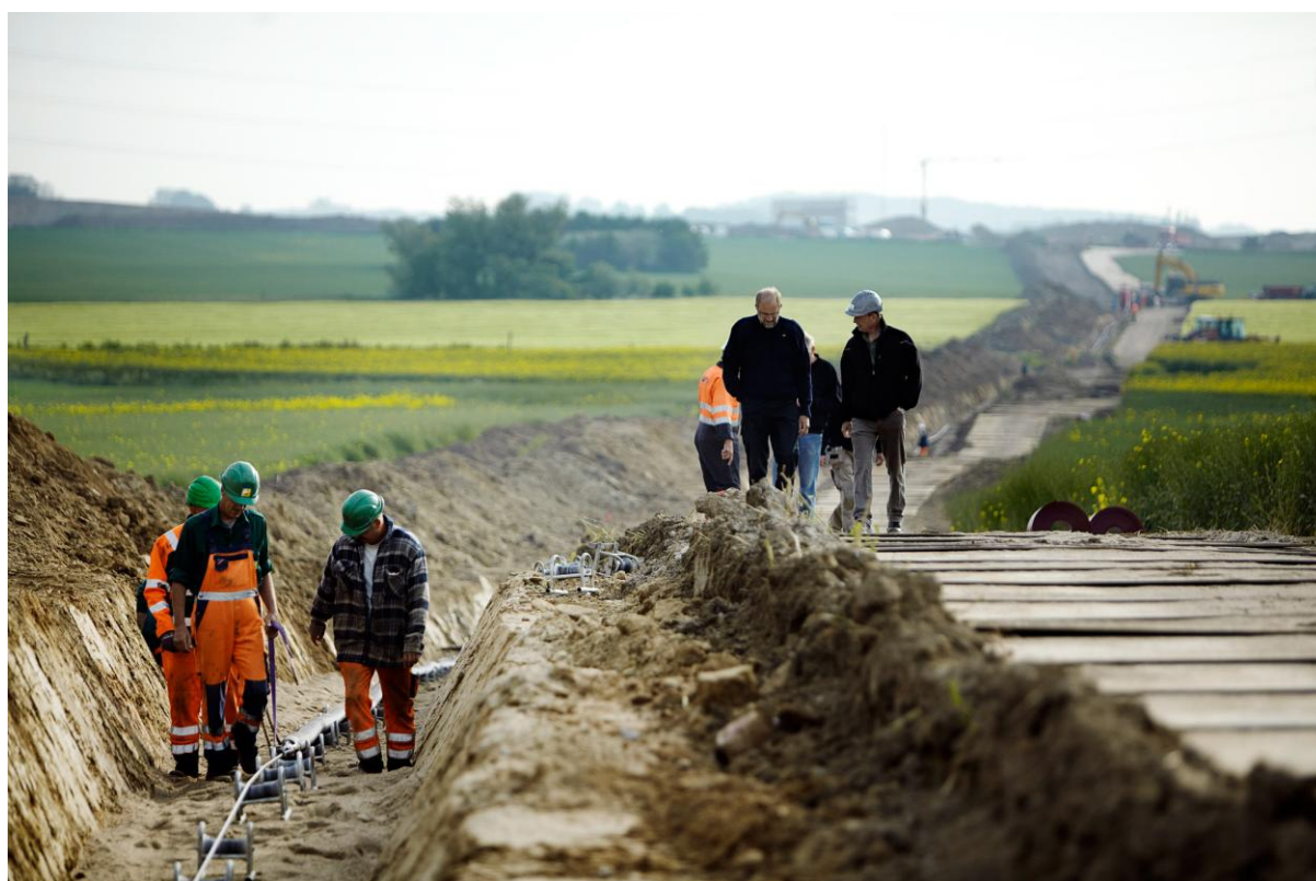
Figure 4.4 Installation of underground grid in Denmark
