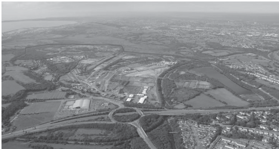
Figure 1 Urban Village site from J43 on M40 with Crymlyn Bog in the distance.
