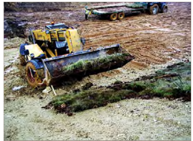
Figure 8. Turfs were also transported by a flat-bed trailer and placed by telehandler
