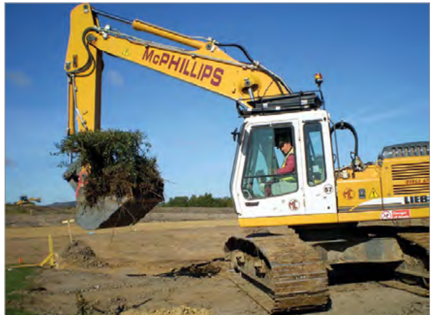
Figure 2. Moving a 1 m section of hedgerow at Lightmoor in September 2007
