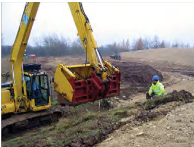
Figure 7. Placing turfs on the new landscape bund at Boston Spa
