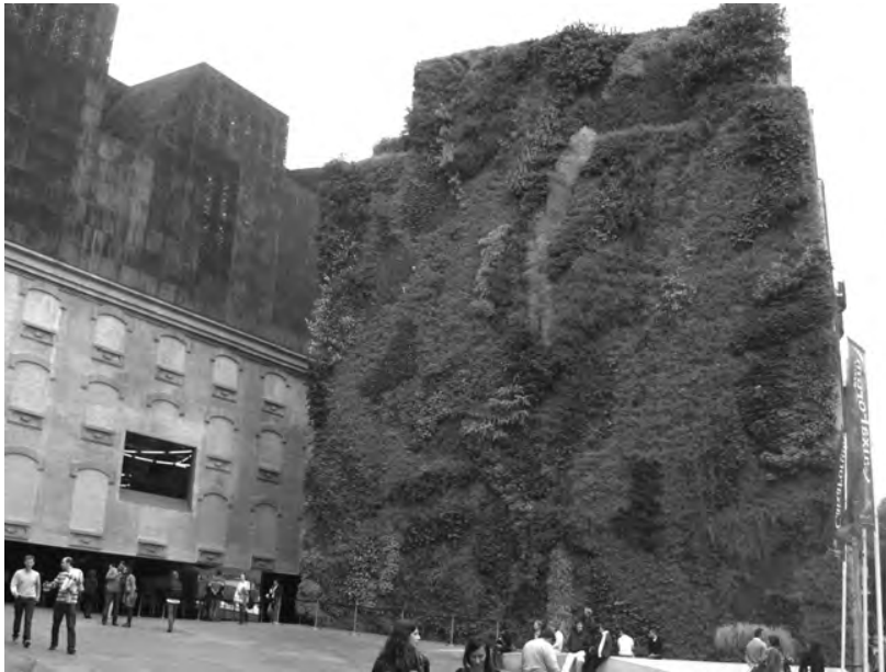
Figure 5.6.2 The 'green wall' at the CaixaForum culture forum on the Paseo del Prado in Madrid, which covers some 460 m 2 and supports 15,000 plants from 250 different species. Copyright: John Box (author)
