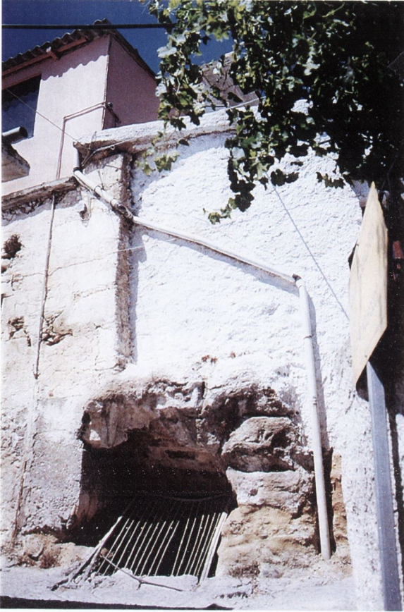
A Polyrhennia: shaft off village street
