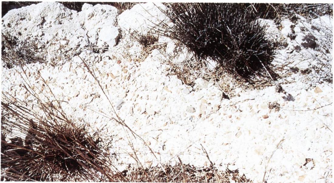
C Kouphonisi : opus signinum of aqueduct 2 of water system 2
