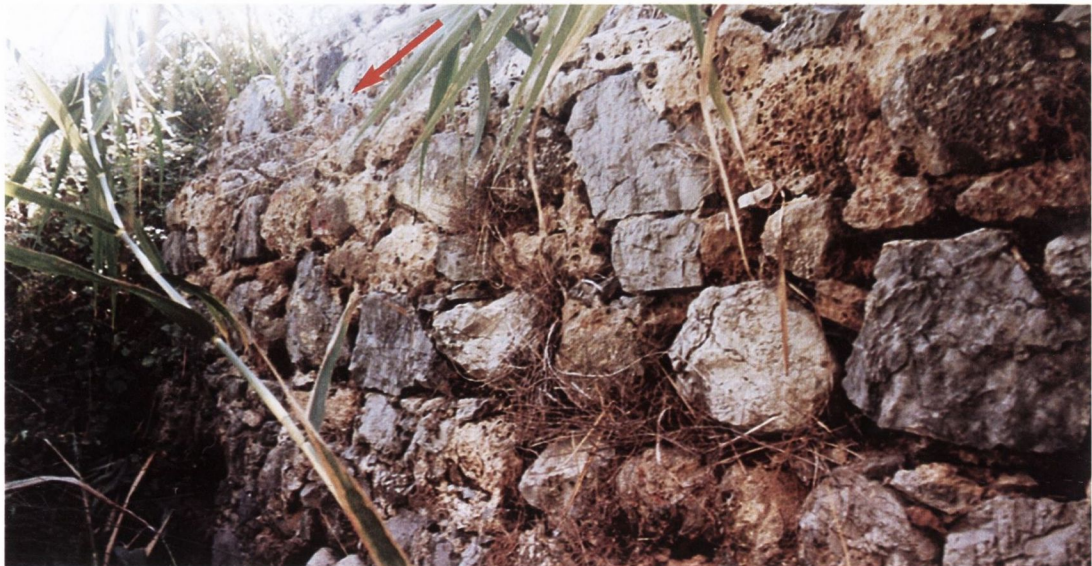
C Malia : stonework of cistern
