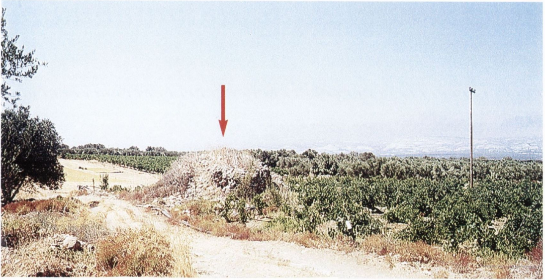
A Pyloros : collapsed and badly damaged structure
