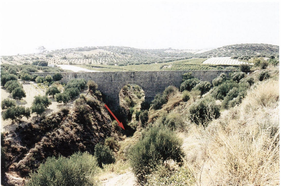
B Knossos : Venetian aqueduct bridge crossing the Vlychia River
