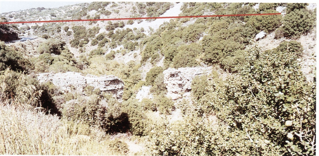
C Chersonisos : free-flow bridge of Xerokamares 2 The red line shows the original height of the bridge
