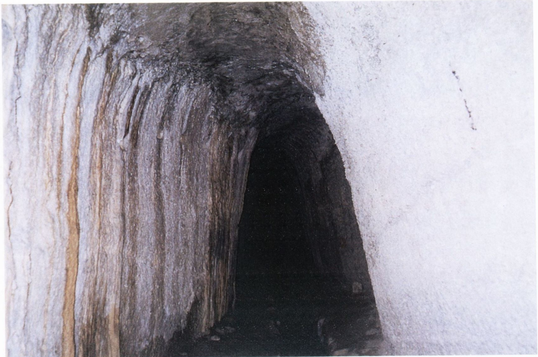
A Eleutherna : rock-carved aqueduct, photographer facing west
