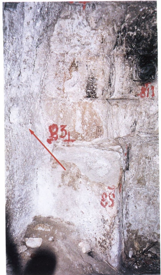
C Eleutherna : back wall of rock-carved aqueduct, lamp niche indicated by the arrow
