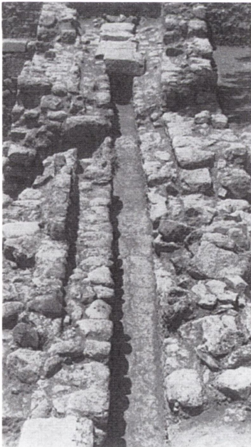
B Knossos : aqueduct branch supplying the area of the North House (after Sackett et al. 1992, 47, pl. 40a).
