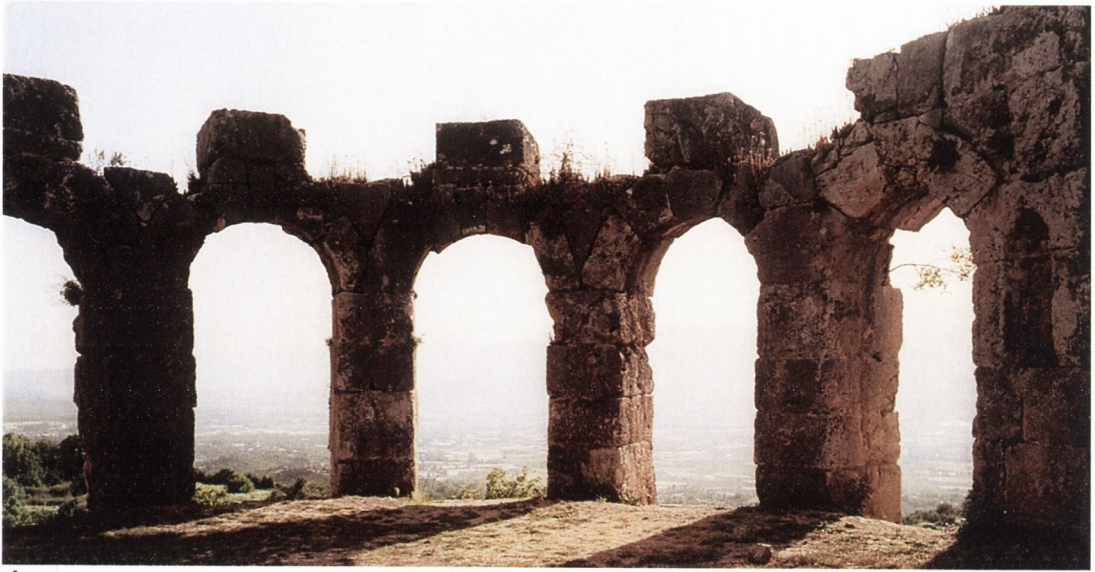
A Tlos: windowed apse in Bath B
