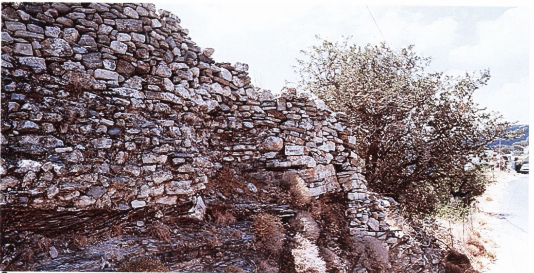
C Elyros : aqueduct
