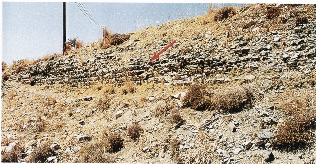
A Lebena : aqueduct AA
