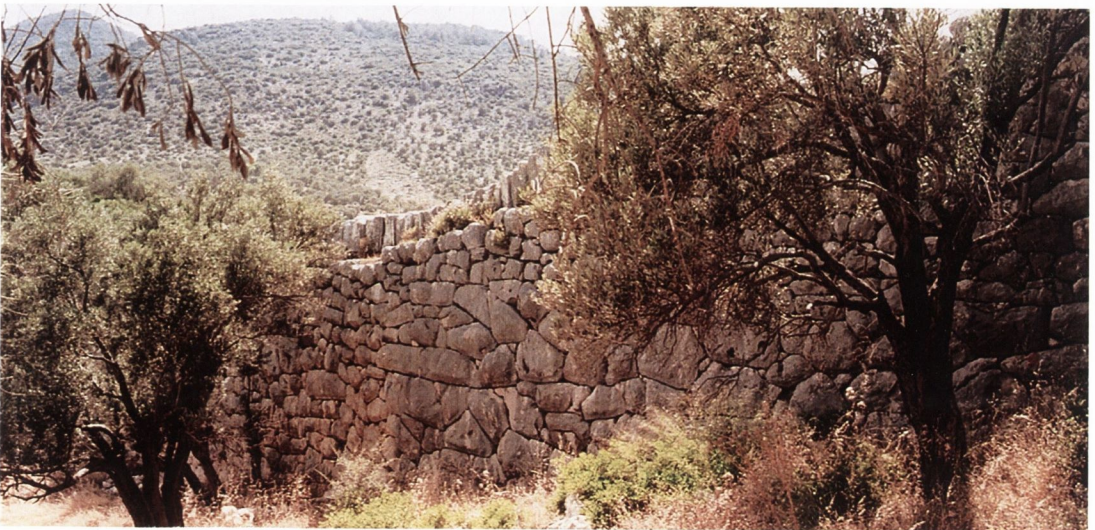
C Patara siphon: polygonal substructure
