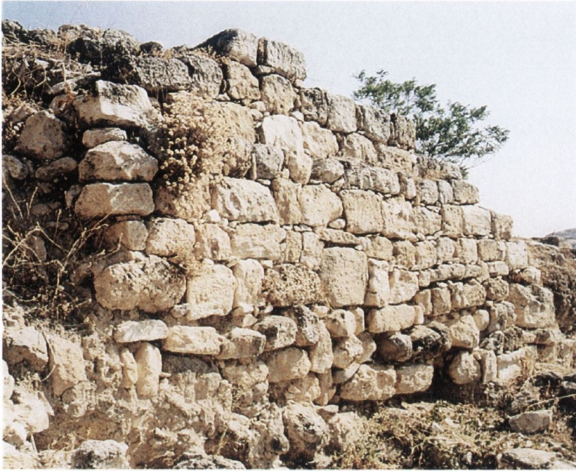
A Knossos : elevation of aqueduct branch in North House
