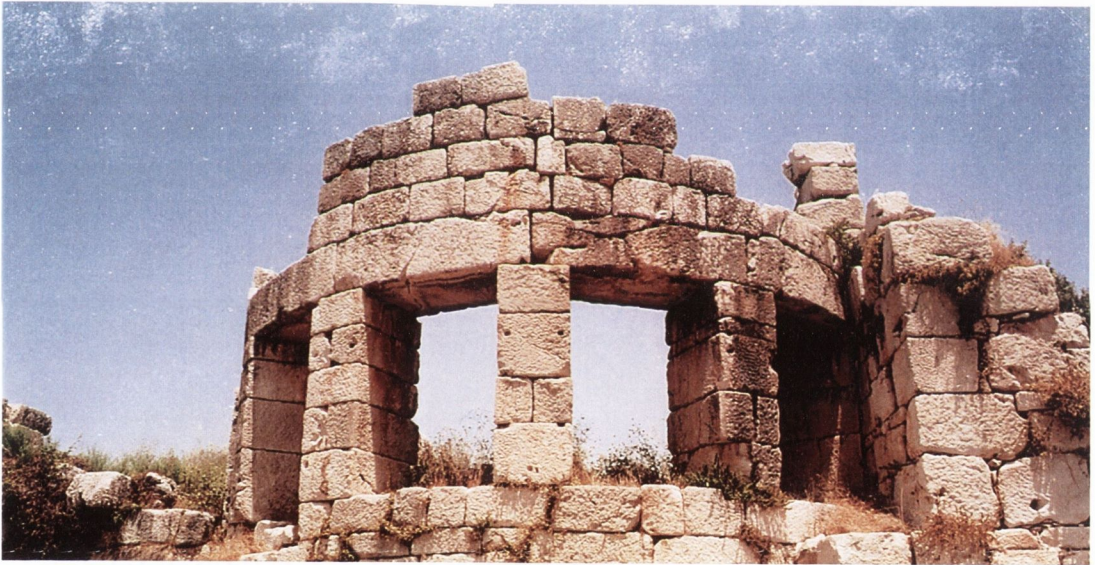
B Patara: windowed apse in the North Baths
