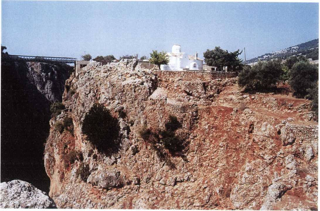
A Aradena : bridge over ravine entering the village
