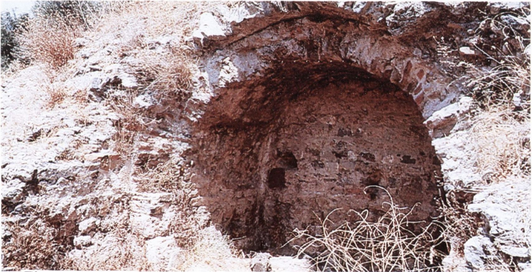
B Elyros : vaults of the cisterns
