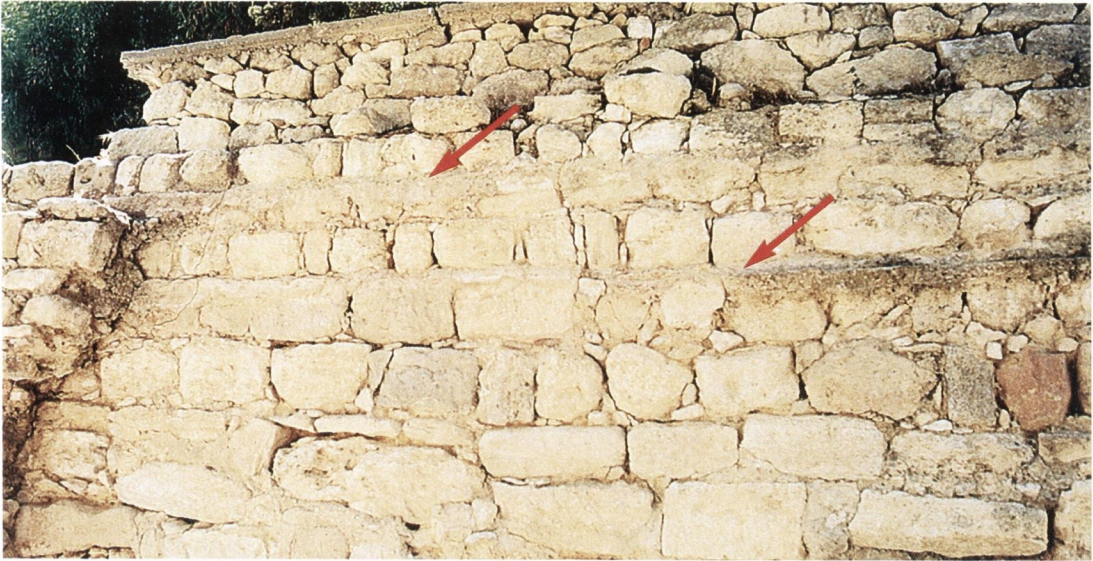
A Knossos : opus signinum visible in side of Royal Road indicating piping
