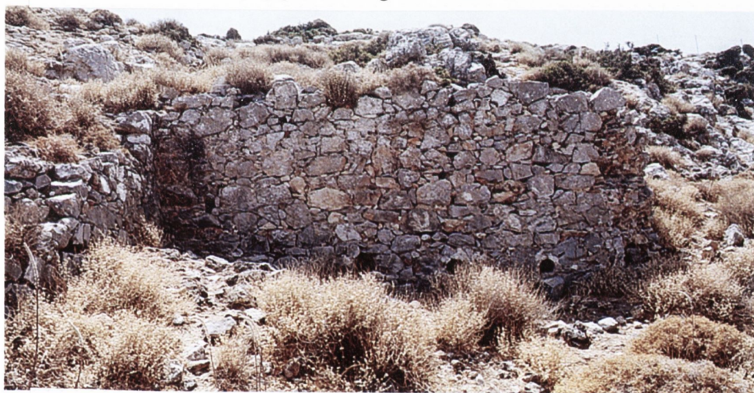
B Diktynnaion Sanctuary: wall with pipes
