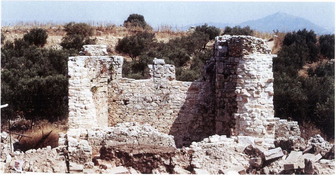
A Aptera: Bathhouse to the north of triple cistern
