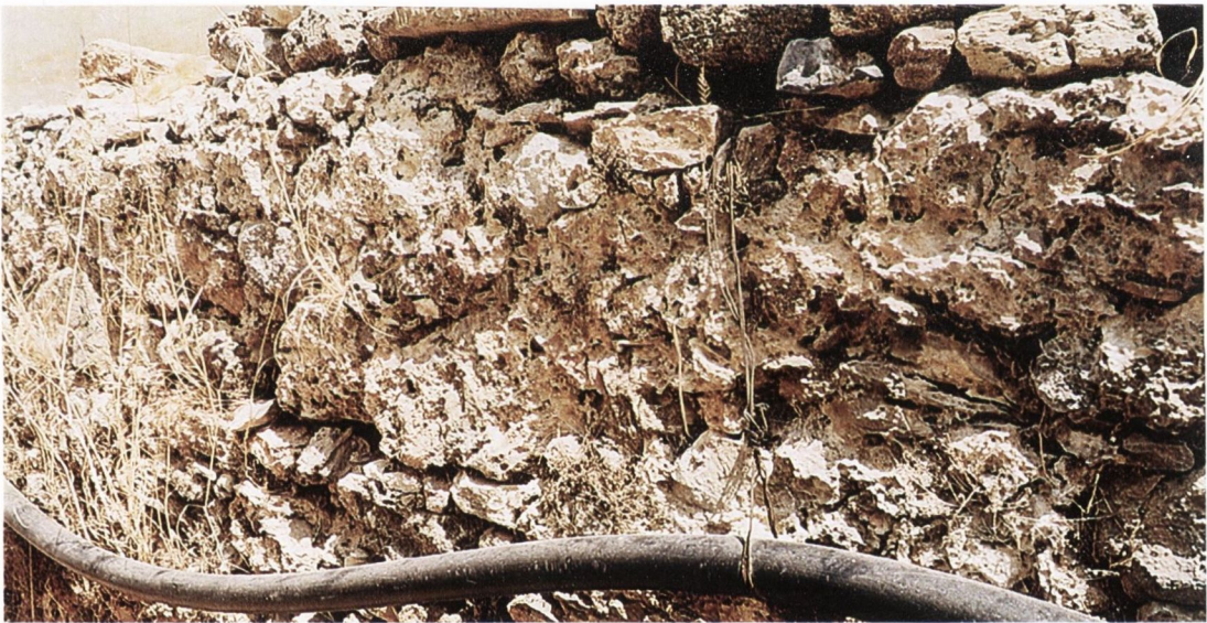
B Phalasarna: substructure of aqueduct
