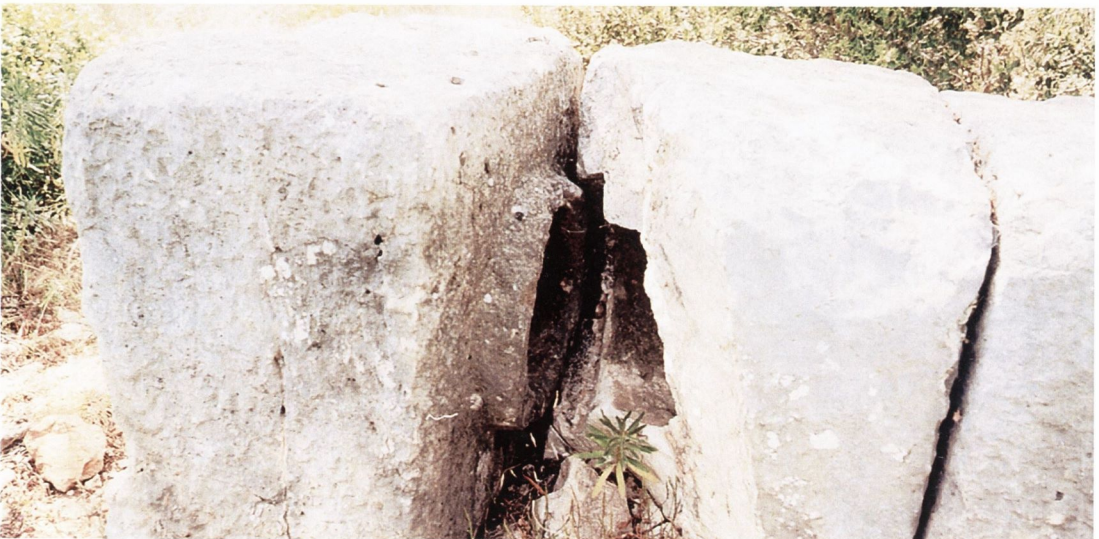
C Patara siphon: detail of stone pipes
