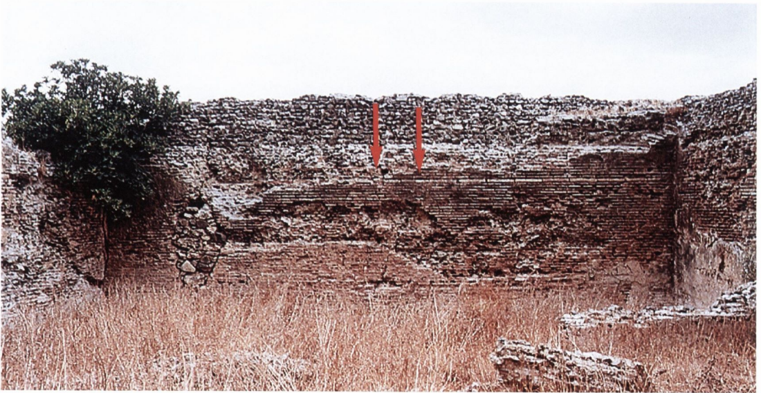
C Kastelliana : north wall with evident bonding course
