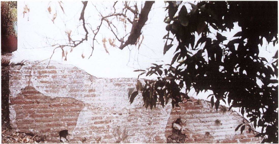
A Lappa: brickwork in the foundations of chapel of Aghios Nikolaos
