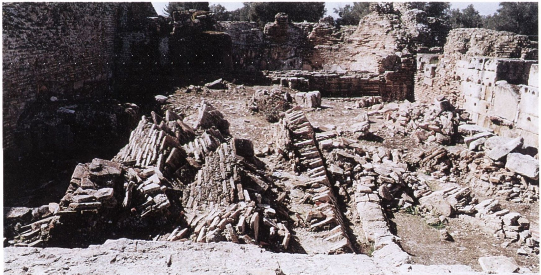
B Gortyna: Praetorium Baths, collapsed vault in caldarium 13
