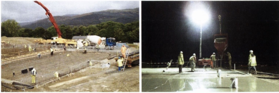
Fig. 7.8: PenyCefn Treatment Works Construction
