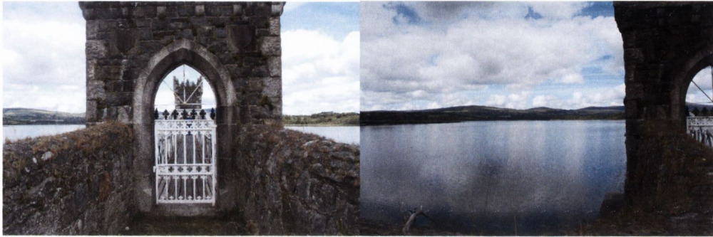
Fig. 7.2: Draw-off tower at the Lower Vartry Reservoir (L); Vartry Reservoir (R)
