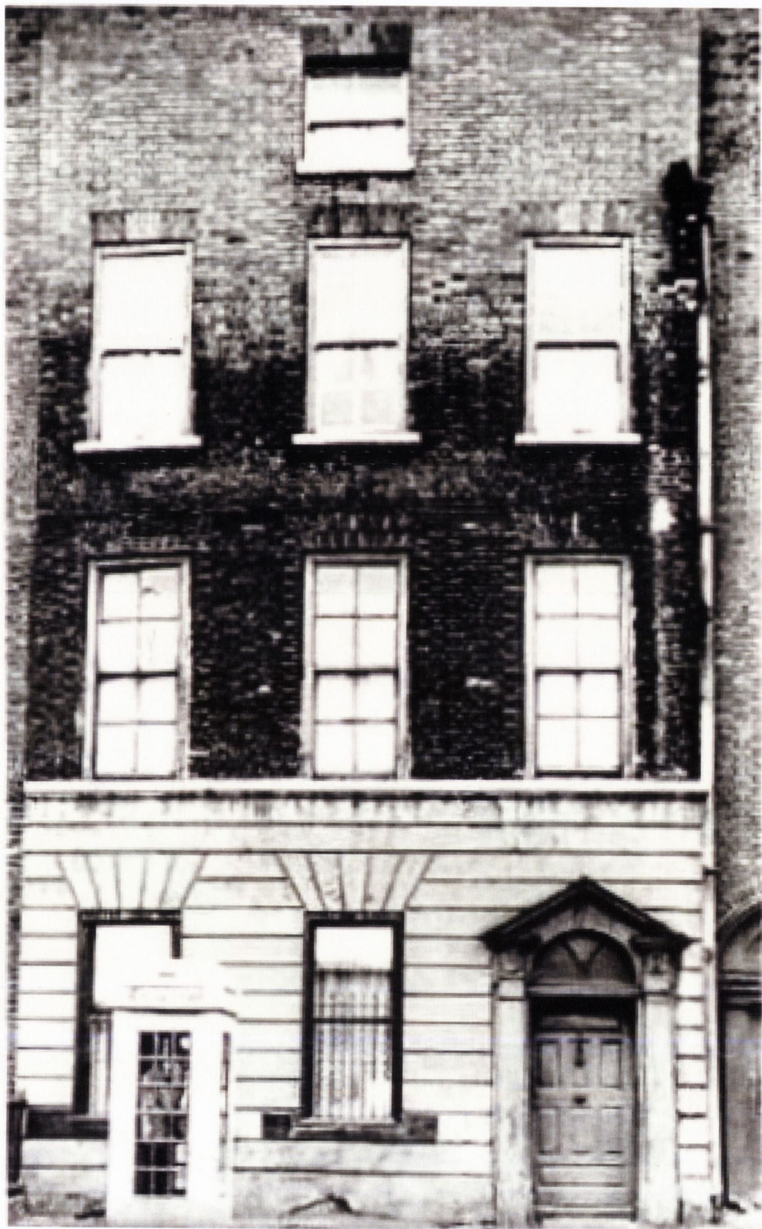
Fig.2.1. Kilkenny marble downpipe to the right of doorway on Stern Tighe's house, Usher's Quay, Dublin. Courtesy Irish Architectural Archive.
