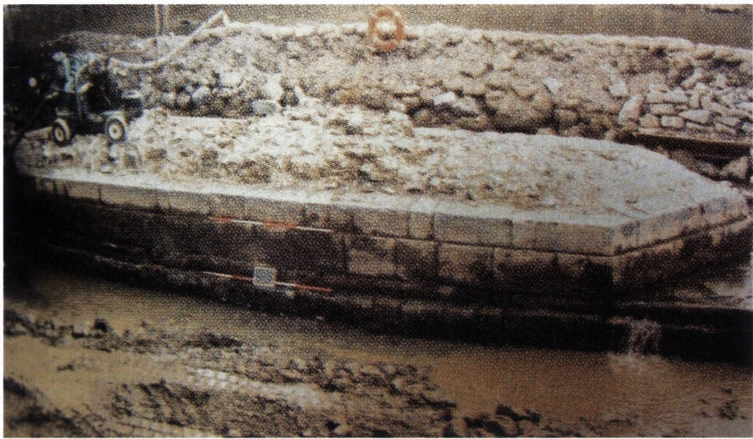
Fig.5.5. View of exposed ashlar of Kilkenny marble used in the foundation of the post 1763 John's Bridge. Source: Ian Doyle, 'The lost bridge of Kilkenny City: John's Bridge, 1765-1910', in Archaeology Ireland , Spring 2003.
