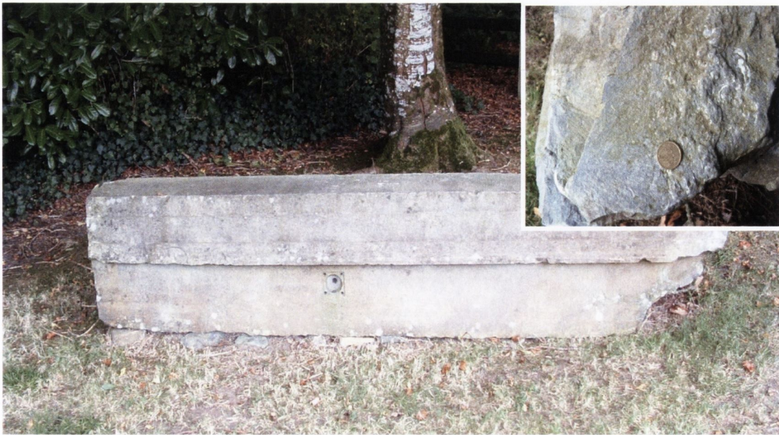
Fig.6.12. Part of doorframe at Castle Morres. Fossilisation clearly visible in detail photo inset.
