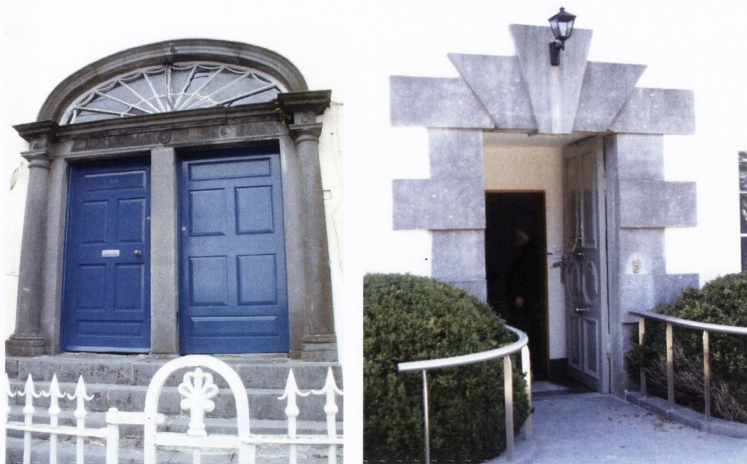
Figs.6.15 & 6.16. The double doorcase of Kilkenny marble on The Bridge House, Kilkenny, contrasted with the Gibbsian style of the Bishop's Palace.
