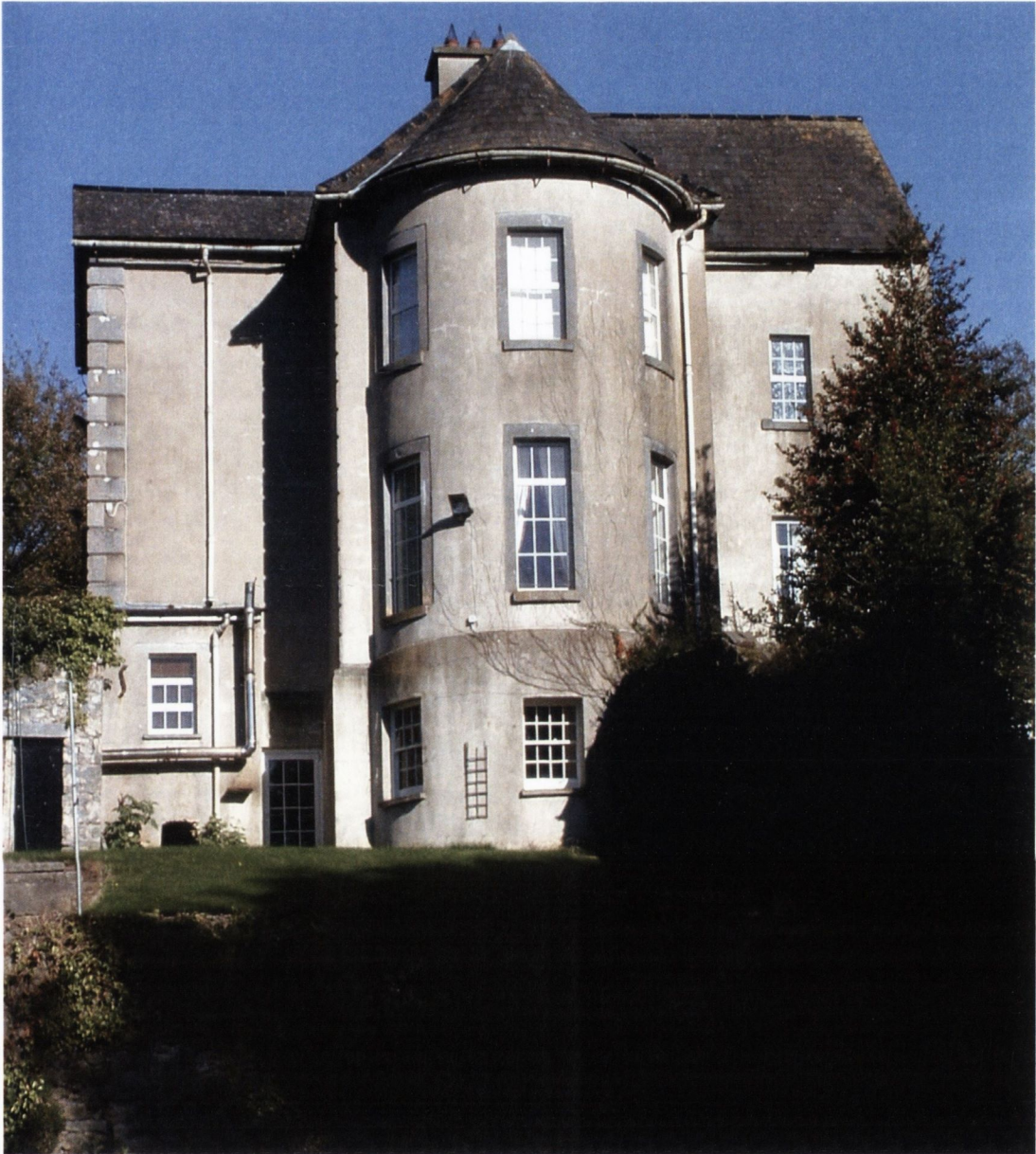
Fig.6.23. Millmount House, Maddoxtown, Co. Kilkenny. Full height basement visible on the west side facing the river Nore.
