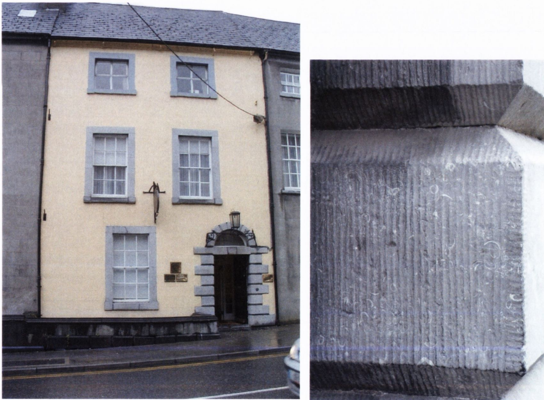
Figs.6.13 & 6.14. Colles House on Patrick St. with detail of delicate chisel work on chamfered door surround.
