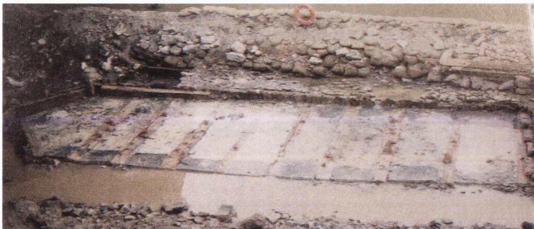
Fig.5.4. The foundation of one of the piers of John's Bridge, as constructed by William Colles. Source: Ian Doyle, 'The lost bridge of Kilkenny City: John's Bridge, 1765-1910', in Archaeology Ireland , Spring 2003.
