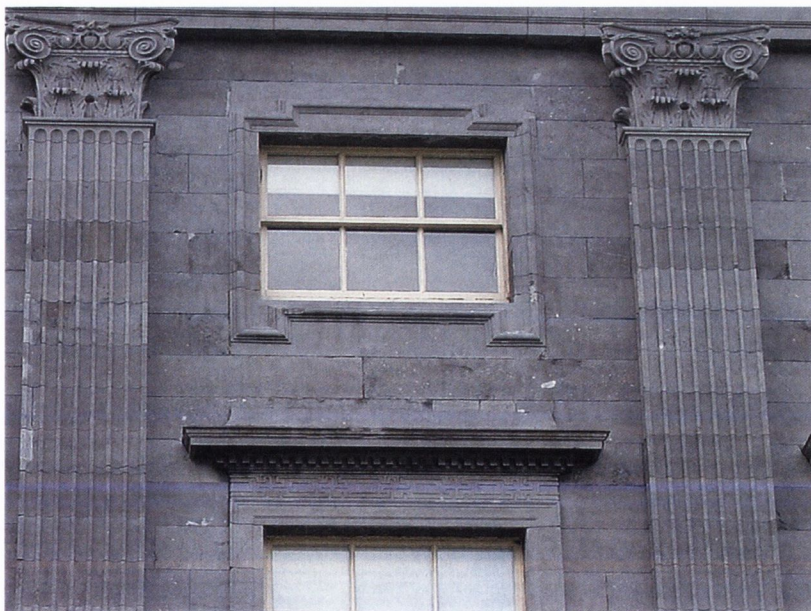
Fig.5.10. Detail of river front of the Custom House, now the Hunt Museum, in Limerick. The dark grey/blue colour with white circular fossils is consistent with the appearance of Kilkenny marble.
