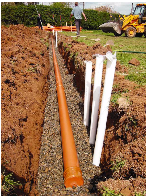
Figure 3.3. Construction of percolation trench.
