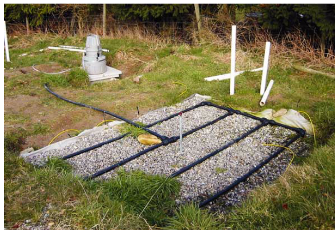
Figure 3.7. Completed stratified sand filter on Site 4.
