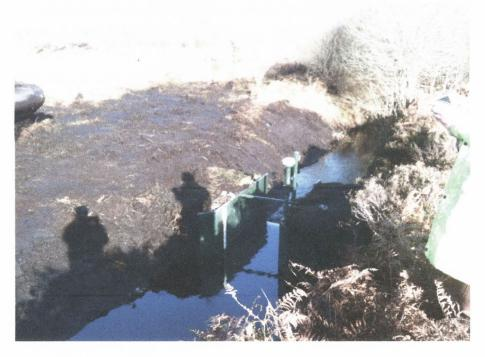
Figure 4.10. EPA Weir installed in drain TD2
