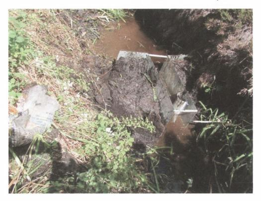
Figure 4.14. FB2 Flume installed in the FB2 Drain (note: stilling well and staff gauge later installed upgradient of flume).
