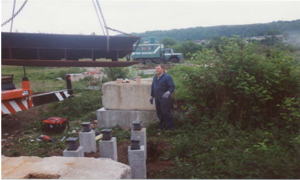
Figure 4-2 Lowering of the pile cap onto TG3
