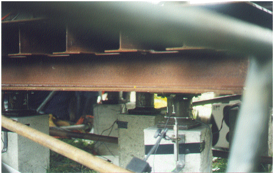
Figure 4-4 Load cell fixity to pile head (top left), Load cell-pile cap welded connection (top right), Assembled test setup (bottom)
