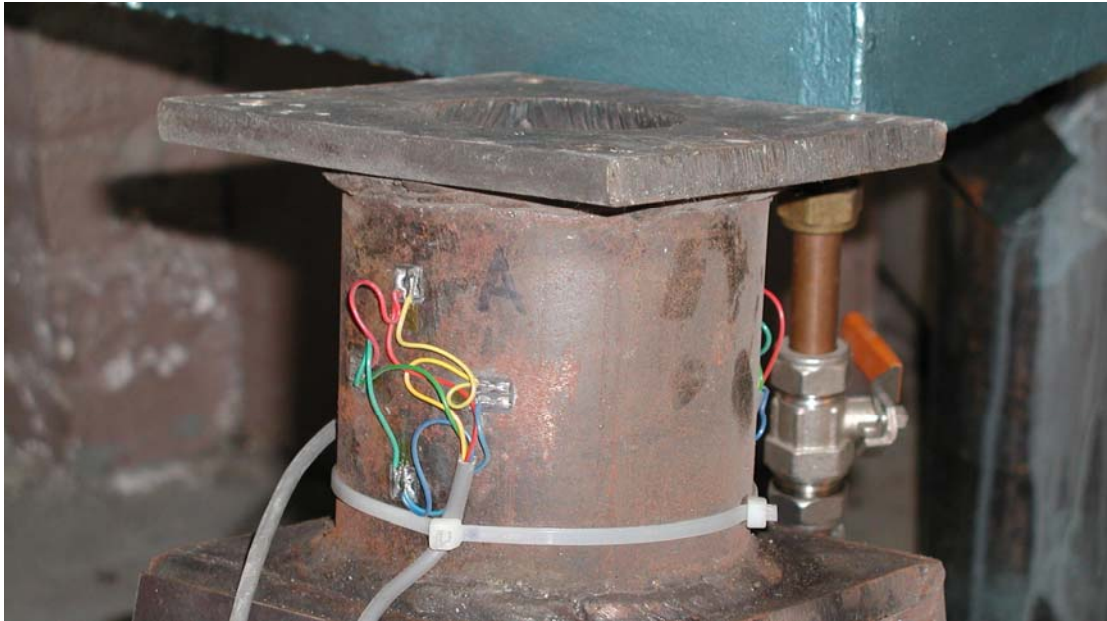
Figure 4-3 TCD Pile head load cell
