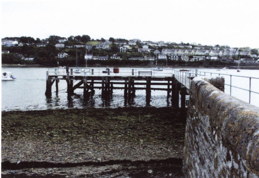
Figure 6.16 View of the structure at ground level.
