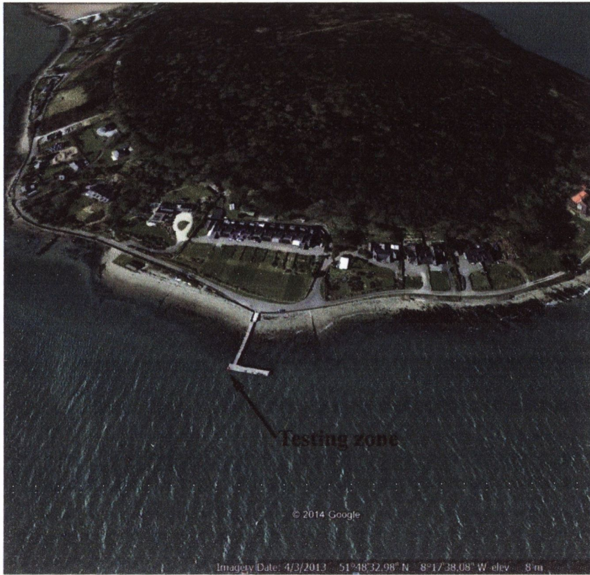
Figure 6.15 Aerial view of testing zone in Currabinny, Cork Harbour. Source: Google Maps (retrieved 15/09/2014).
