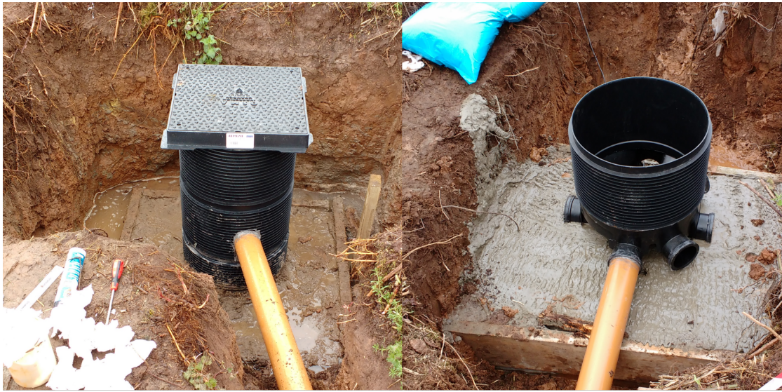
Figure 3.8: The Armagh Observatory permanent magnetometer installation. Left: the inspection chamber which housed the magnetometer before being buried. Right: the inspection chamber which housed the data logger.
