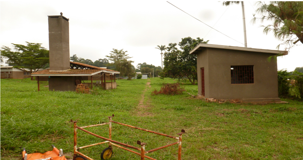
Non-functioning incinerators, Kigadi Hospital, Kibaale District 2014 Source: Researcher (DO, P6)
