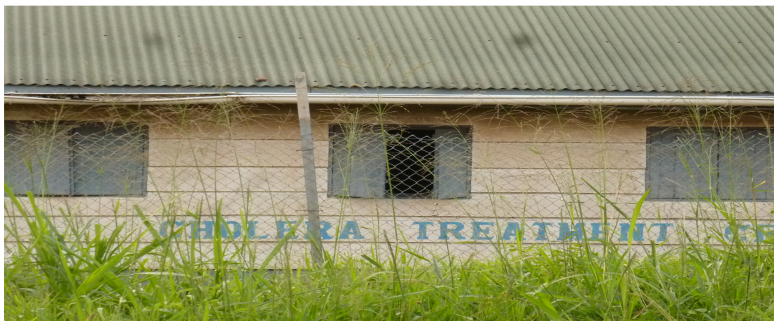
Cholera Isolation Unit, Bundibugyo Hospital
