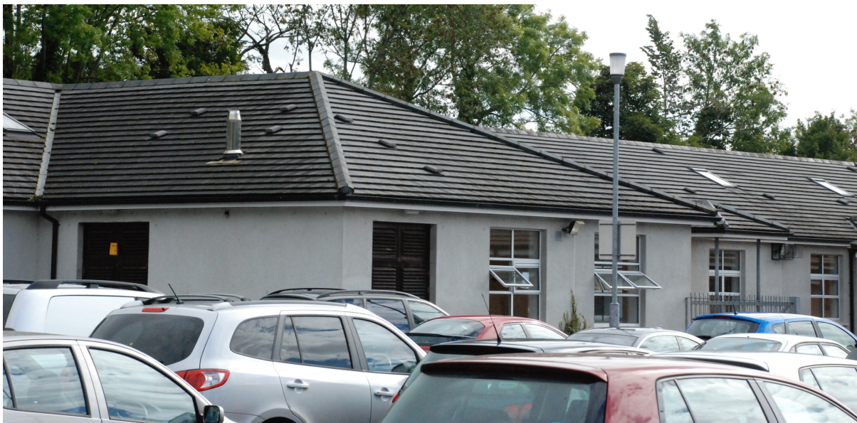
Figure 7.1 Research School Exterior A
