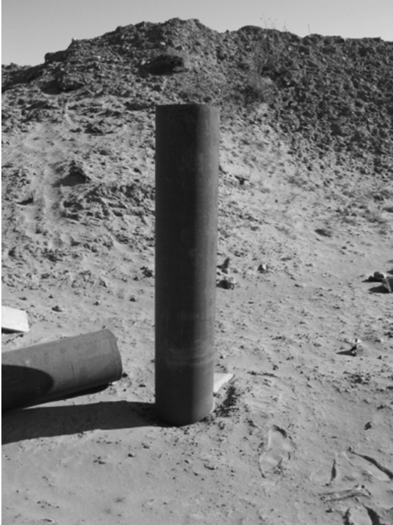
Figure 2. Installed pile at test location.
