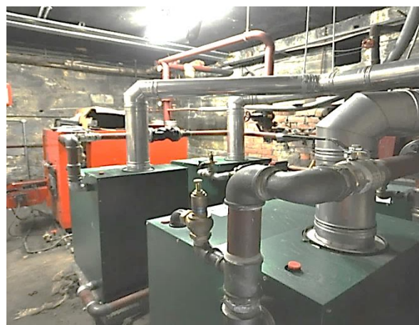
Figure 5.82 - New oil boilers being installed in Letterkenny cathedral
