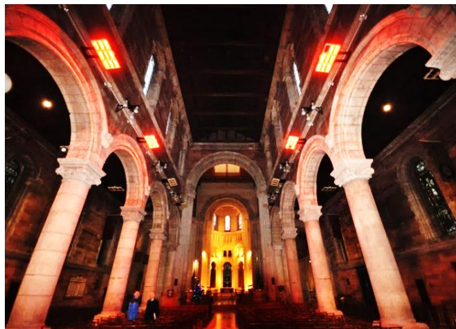
Figure 5.20 Electric radiant heaters switched on in St. Anne's cathedral
