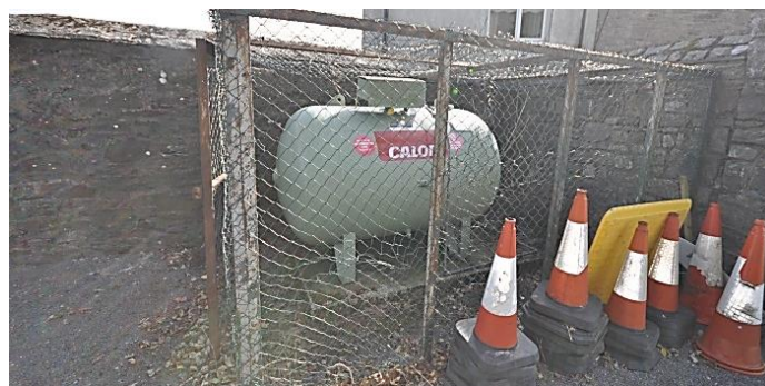
Figure 4.27 - St. Brigid's cathedral Kildare, gas storage tank
