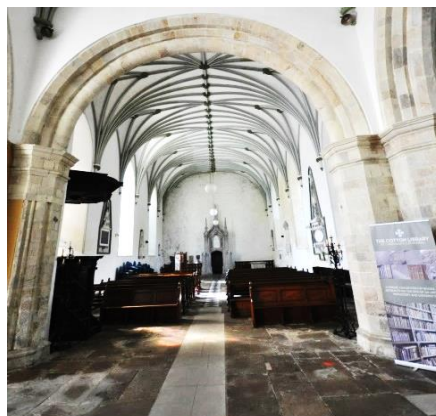
Figure 5.95 – Lismore cathedral showing stone floor and area of the nave usually not used
