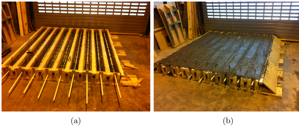
Figure 6.9.: Concrete beam casting; (a) formwork; (b) concrete poured into mould
