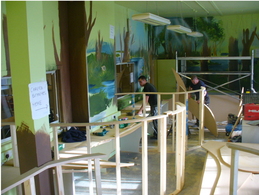
Figure 3.22 Construction of the Team Space
