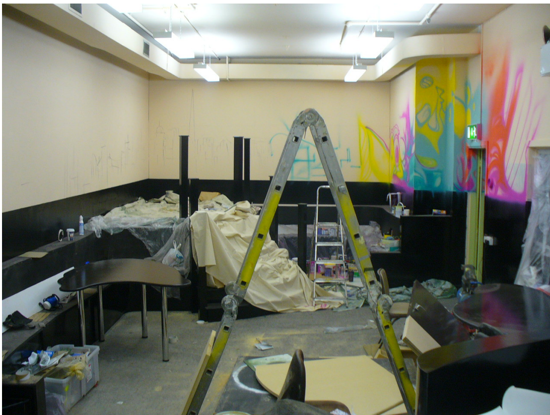
Figure 3.23 Construction of the Ideas, Breakout and Presentation Space
