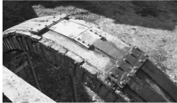
Figure 2. Arch after intervention using Borri and Castori's system [3].
