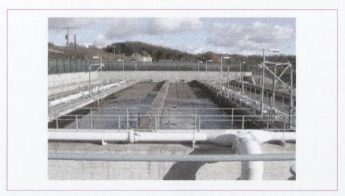
Figure 9. 8 Photograph showing the extended aeration process of Leixlip WwTW
