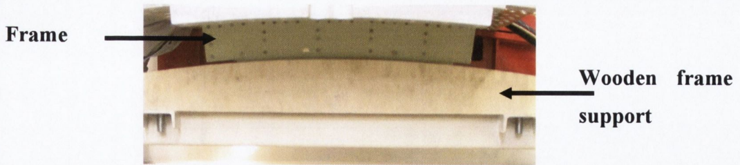
Figure 3.6 Frame inner flange wooden support
